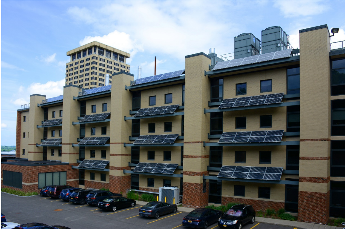
Baker Laboratory 25 kW solar photovoltaic array that also provides window shading for the building’s south side
