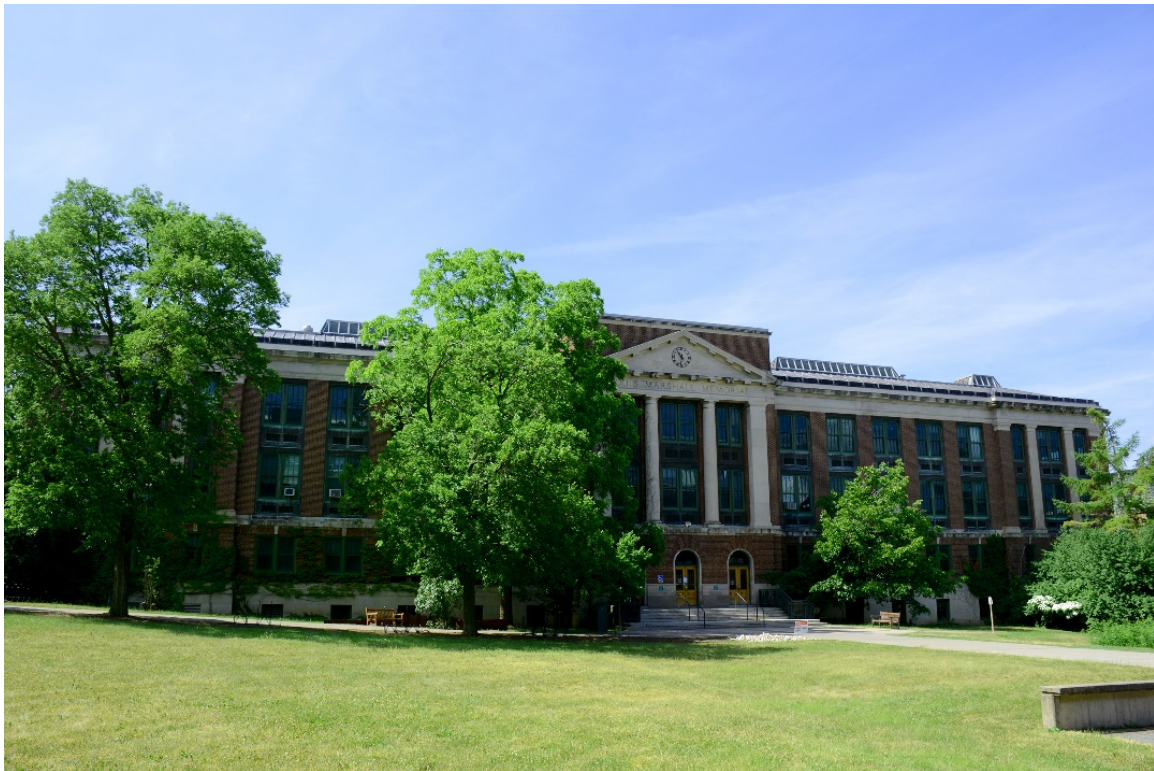
Marshall Hall – Full renovation planned through 2022; discontinued steam use and designed to achieve SUNY goals for Deep Energy Retrofits (DER)
