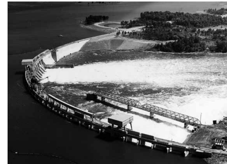
Long Sault dam (left) during the construction of the Moses-Saunders power dam (right).
