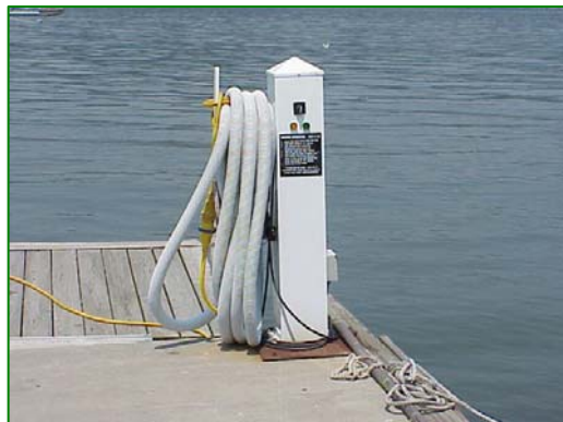
A boat pump-out unit installed in 2000 located at the Coney Island WPCP, Source: NYCDEP Boat Pump Out Remote Unit.
