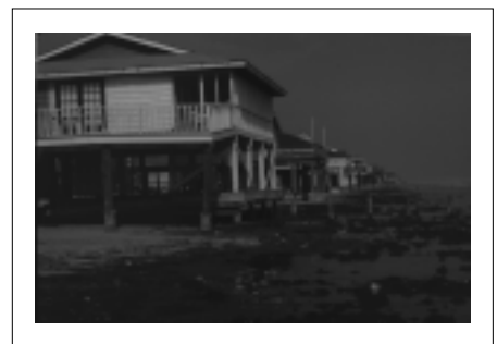
FIGURE 35 Erosion Damage from Tropical Storm Frances (1998)
