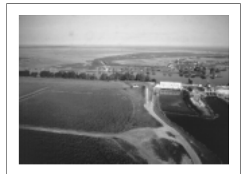
FIGURE 2 Water Control Structure
