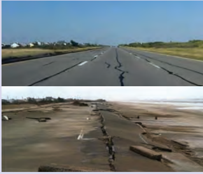
Figure L-11: Ocean Parkway before and after Sandy. If dunes were not there, more damage may have occurred. (NYSOPRHP, 2012)
