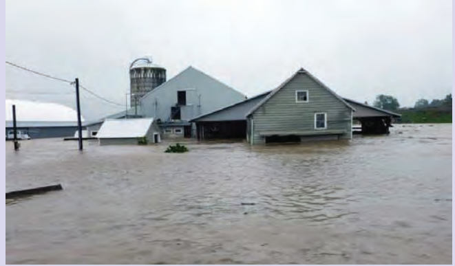
Figure L-02: Floodwaters from Irene inundate dairy barn at Maple Down Farms II. (NYS Responds Report, 2012)
