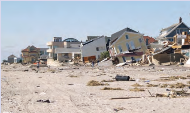
Figure L-03: Building damage in the Rockaways. (NYS DOS, 2012)
