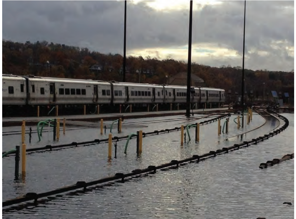
Figure T-11: Flooding at Metro-North's Harmon Yard in Croton-on-Hudson exemplified the challenges faced by Metro-North employees in restoring service after Superstorm Sandy. (MTA Metro-North Railroad, 2012)
