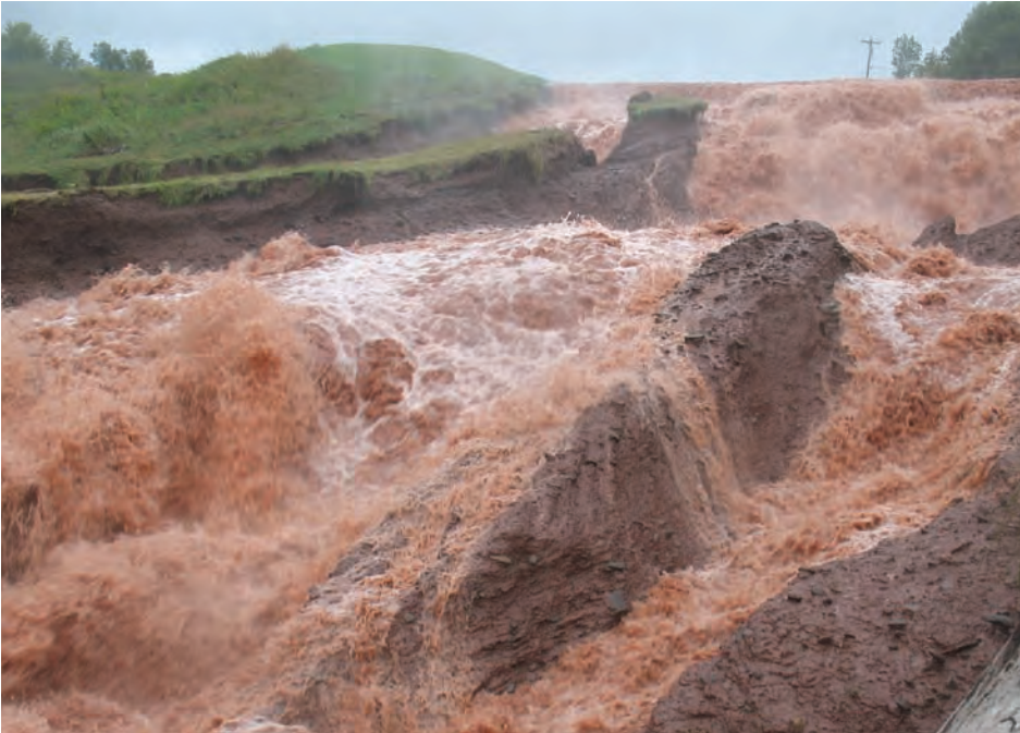
Figure L-25: Batavia Kill Dam No. 1 with flow through emergency spillway eroding downstream bank during Irene (NYSDEC, 2011)
