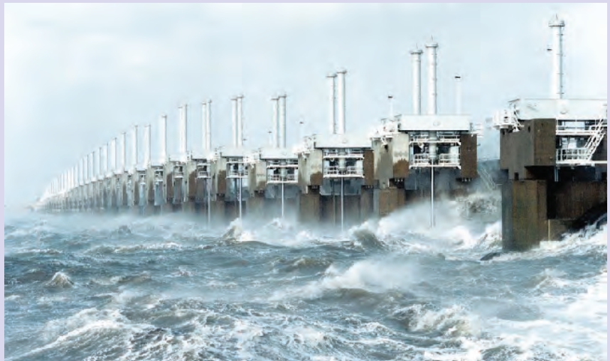
Figure L-16: Eastern Scheldt storm surge barrier in the Netherlands. (Delta Works Online, www.deltawerken.com )
