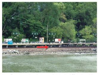
Notes: The red arrow shows the lowest critical elevation, LCE=6.6 feet, of the rail tracks located in waterway zone Z3=9 feet. The elevated concrete structures are the passenger platforms at an elevation near 11 feet. Note the low-lying parking lot in background.
