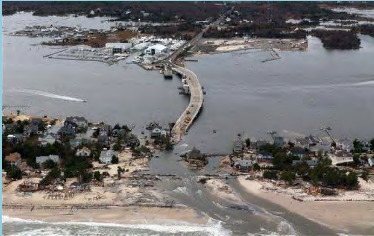
Mantoloking Bridge, Ocean County, New Jersey. New inlet formed as a result of Hurricane Sandy (left, top and bottom). Emergency repairs to roadway and beach – filling the newly created breach – the week after the storm.
