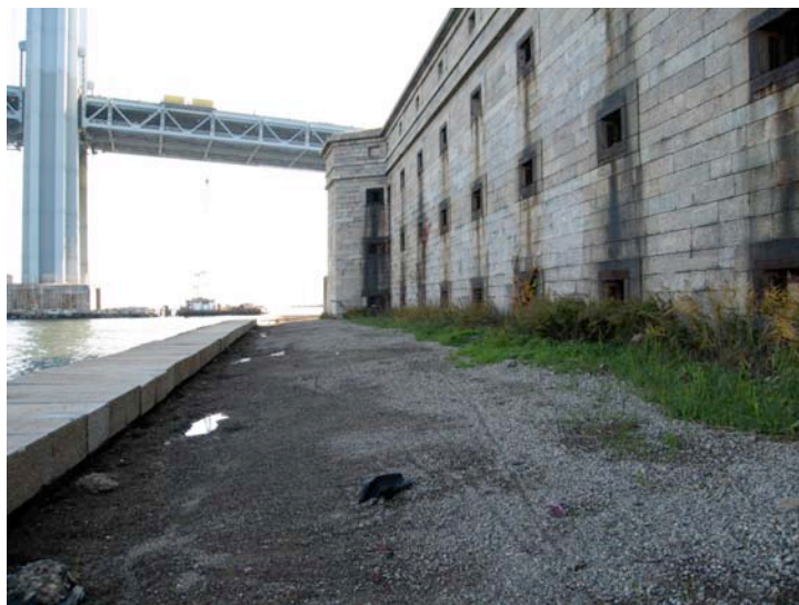
Figure 3.12: The surface of the filled moat consists of gravel and earth and is uneven and puddling in places. SUNY ESF, 2007.
