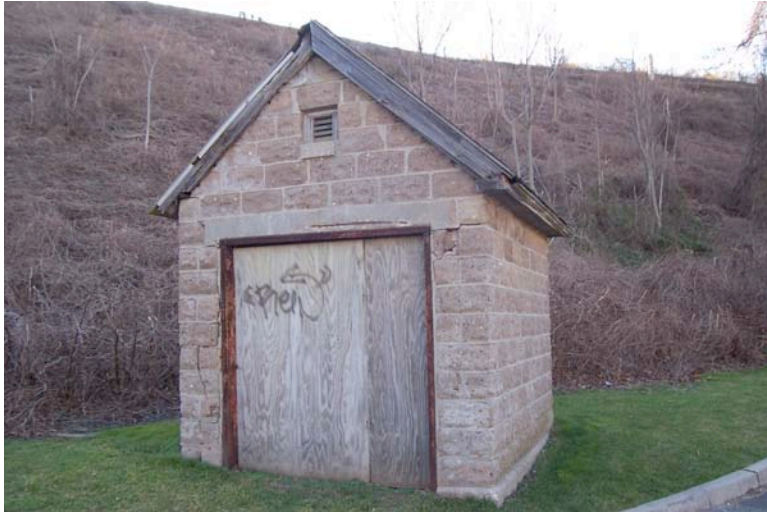
Figure 3.26: The small concrete block building at the base of the slope to the south of the torpedo storage building measures approximately 9 feet by 11 feet. SUNY ESF, 2007.
