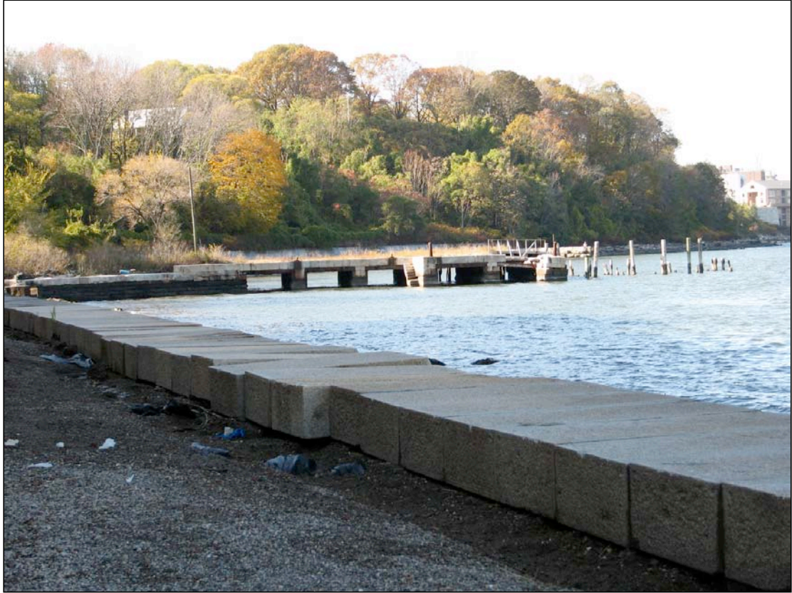
Figure 2.7: The North Stone Dock and Seawall Looking northwest. SUNY ESF, 2007.
