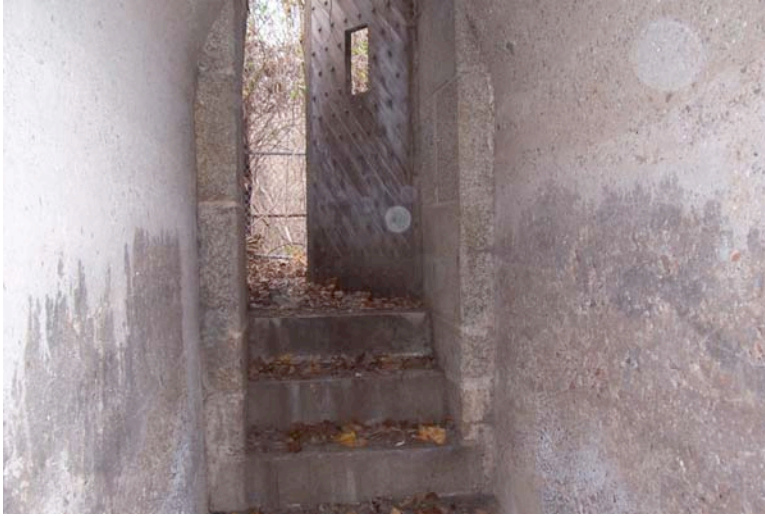
Figure 3.33: A three-inch thick, bronze-fastened, wood plank door with a small vertical window opens outward and leads to steps down into a narrow, barrel-vaulted concrete corridor and interior chamber. SUNY ESF, 2007.
