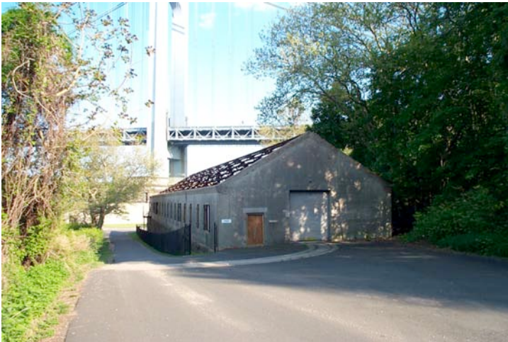
Figure 3.8: Battery Weed Road, measuring approximately twelve feet wide, with the exception of widened areas at the north and south ends of the torpedero storage building, is surfaced in asphalt with some areas of concrete adjacent to the remaining sections of the Mine Railway crossing the road surface. SUNY ESF, 2006
