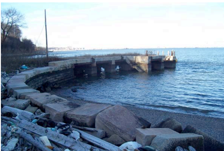
Figure 3.24: A section of the seawall, approximately seventy feet long, to the northwest of Battery Weed has collapsed. SUNY ESF, 2007.
