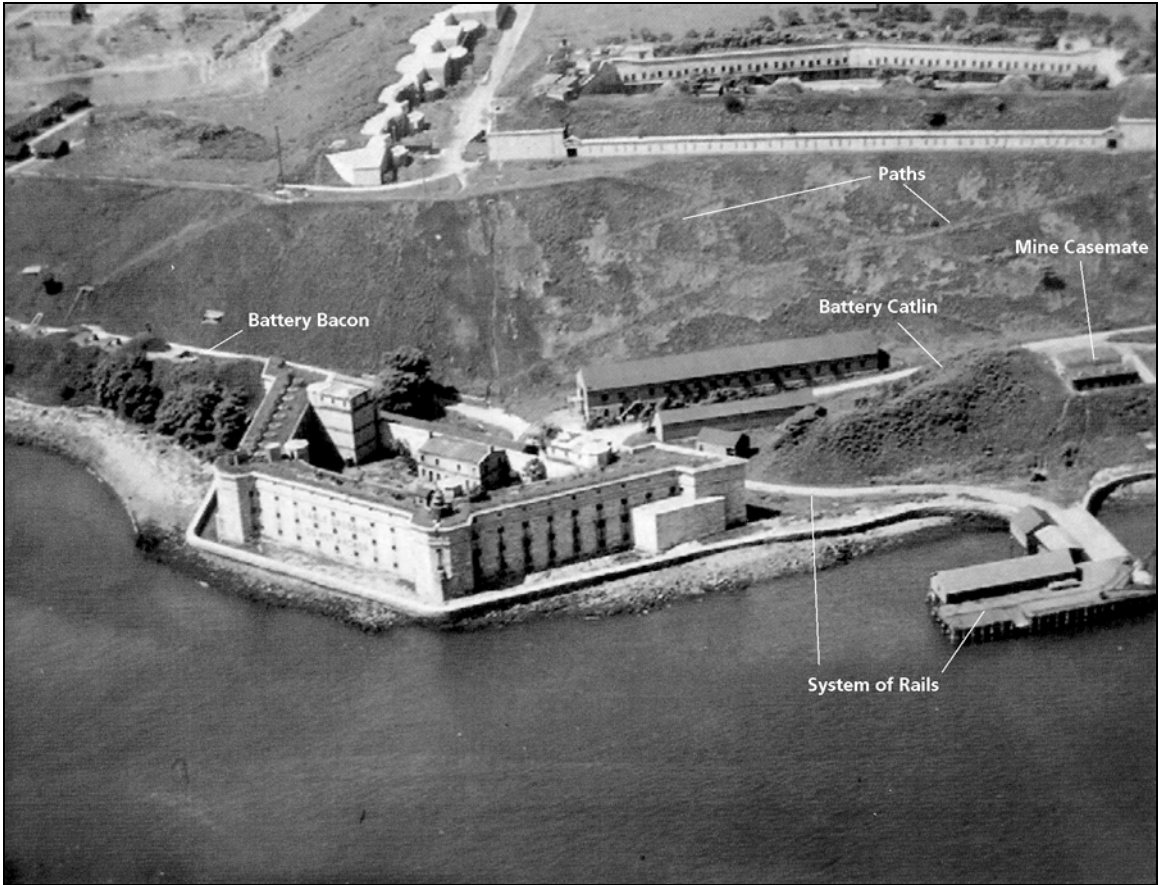
Figure 1.66: An aerial photograph taken from above the Narrows looking toward the west at Battery Weed and the slope above it, 1924. GNRA Archives Photo Collection, 1924, annotated by SUNY ESF, 2007.
