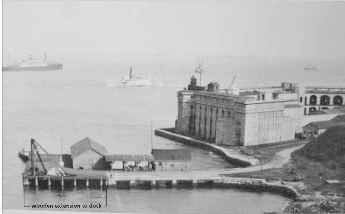
Figure 1.67: Photograph showing the wooden extension and marine crane added to the North Stone Dock. c.1907. Gateway National Recreation Area Archives, Photo Collection, Print #19427, c.1907, annotated by SUNY ESF, 2007.
