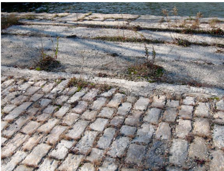
Figure 3.29: The deck is constructed in patterns of small to medium size granite blocks and concrete with steel rails set into the surface along the north side. SUNY ESF, 2007.
