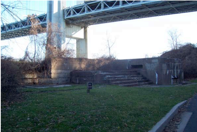
Figure 3.16: The northern end of Battery Bacon consists of a large earth mound measuring approximately 200 feet by 80 feet rising to an elevation of fifty feet above the water level of the Narrows of New York Bay and incorporating concrete walls, steps and gun emplacements. SUNY ESF, 2007.
