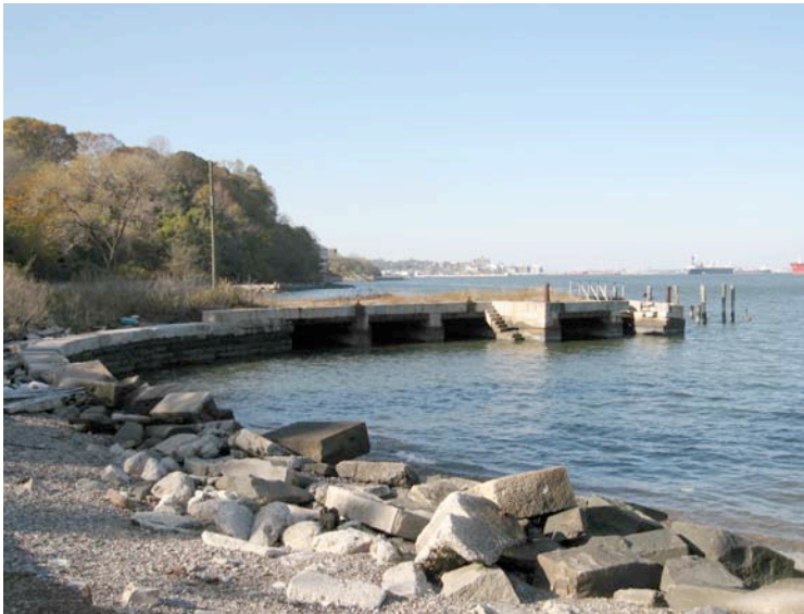
Figure 3.28: The stone dock, extending from the shoreline north of Battery Weed in an L shape, is approximately forty feet wide by eighty feet long. SUNY ESF, 2007.
