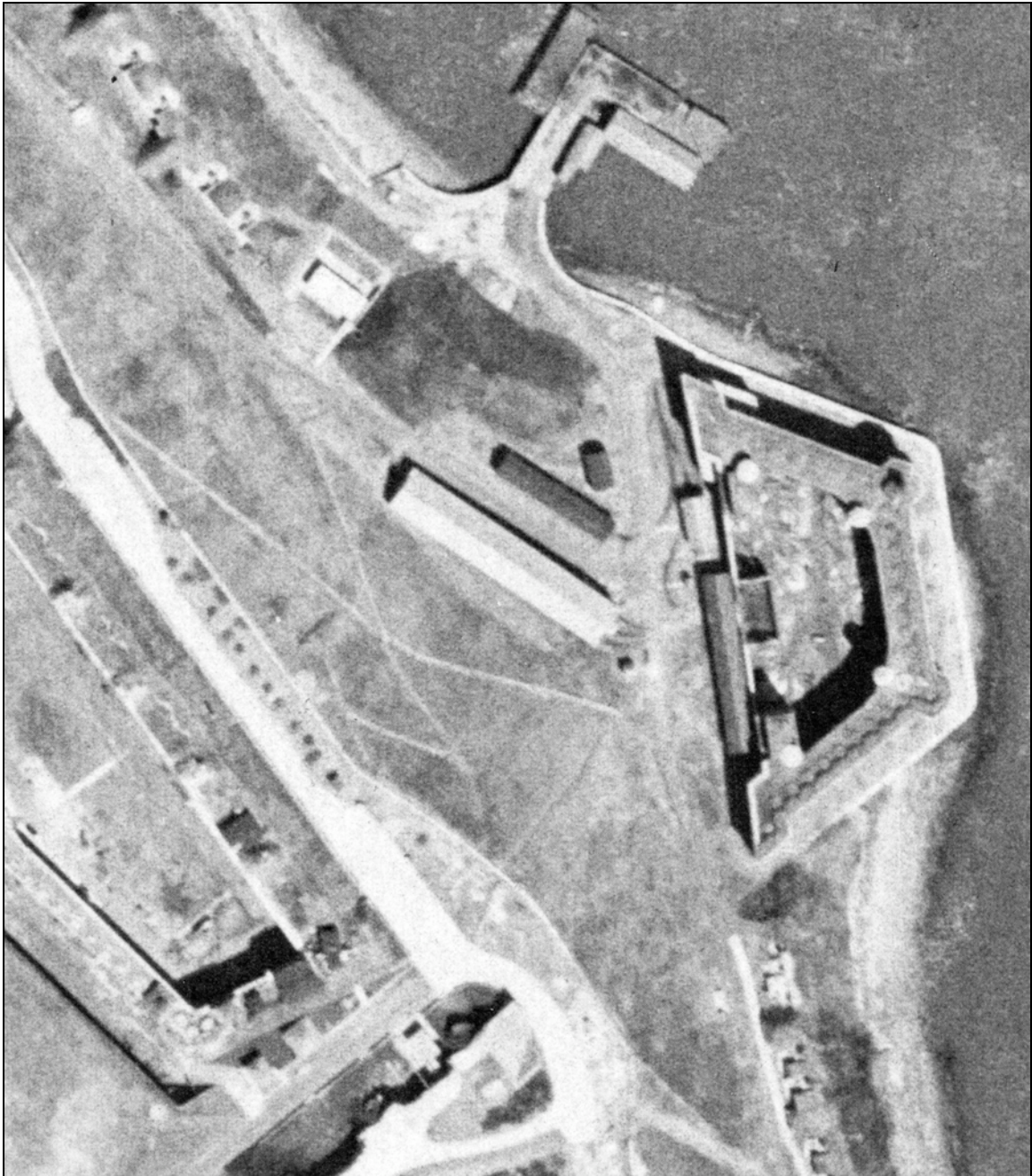
Figure 1.68: Satellite photograph showing Battery Weed at the water's edge, Fort Tompkins, the North Stone Dock with a barge on left, the Torpedo Storage Building and the footings under construction for the Verrazano-Narrows Bridge at lower right, 1940. Pier/Seawall Evaluation and Ferry Feasibility Study, Fort Wadsworth, Staten Island New York, prepared for the National Park Service, 1995, photograph by Aerial Viewpoint Houston, Texas.
