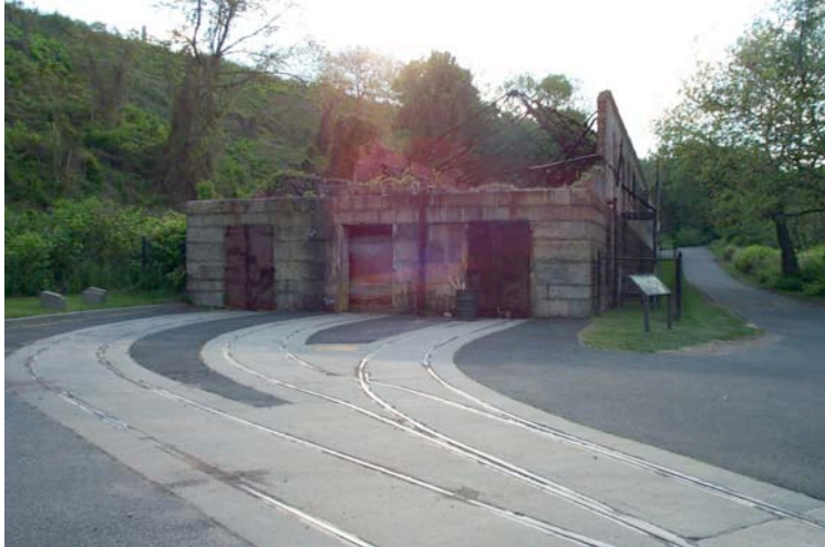
Figure 3.13: The rails set into Battery Weed Road are surrounded with an area of concrete flush with the road surface. SUNY ESF, 2007.
