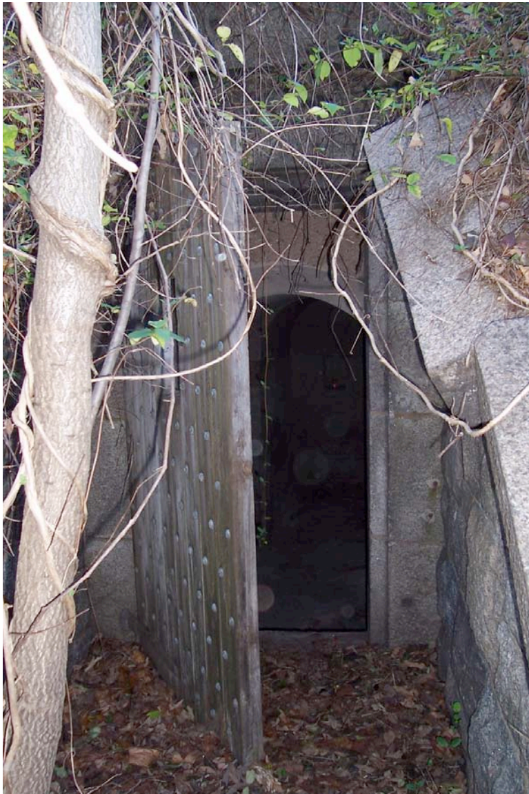
Figure 3.32: One of the granite cap blocks of the entry retaining structure of the Bomb-Proof Parado is heaving probably due to the extensive growth of invasive vines and other vegetation covering the earthwork. SUNY ESF, 2007.
