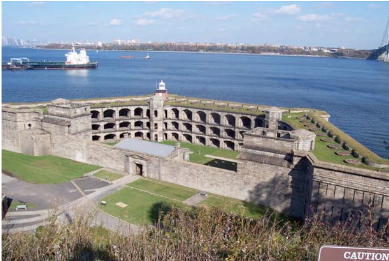
Figure 3.22: Battery Weed, constructed in c.1847- c.1864 of cut granite block, measures 286 feet along each channel front wall, and 450 feet along the west scarp wall. Three casemated tiers, rising one on top of the other, and the fort features a top barbette tier, which is open, and earth covered with a breast height wall, a parapet, along the channel side. SUNY ESF, 2007.
