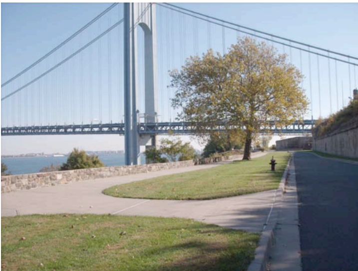
Figure 3.9: Hudson Road, with an asphalt surface, is approximately twenty feet wide and 2,000 feet long running along the top of the slope above Battery Weed immediately to the east of Fort Tompkins. SUNY ESF, 2006
