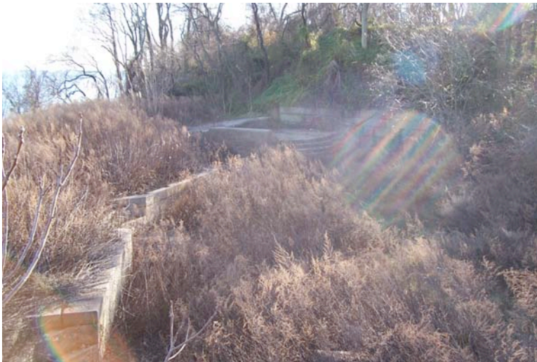
Figure 3.34: Battery Bacon, located just to the south of Battery Weed along the east side of Battery Weed Road, is partially covered in invasive vines, especially over the granite retaining walls and the southern end of the battery. SUNY ESF, 2007.
