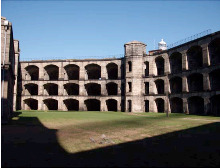
Figure 3.4: The parade ground, measuring approximately 260 feet by 140 feet, is enclosed and framed to the east by three sides of a gently rounded half-hexagon of arched granite casemates with two four-story stair towers and a delicate iron railing between the towers along the top tier. SUNY ESF, 2006
