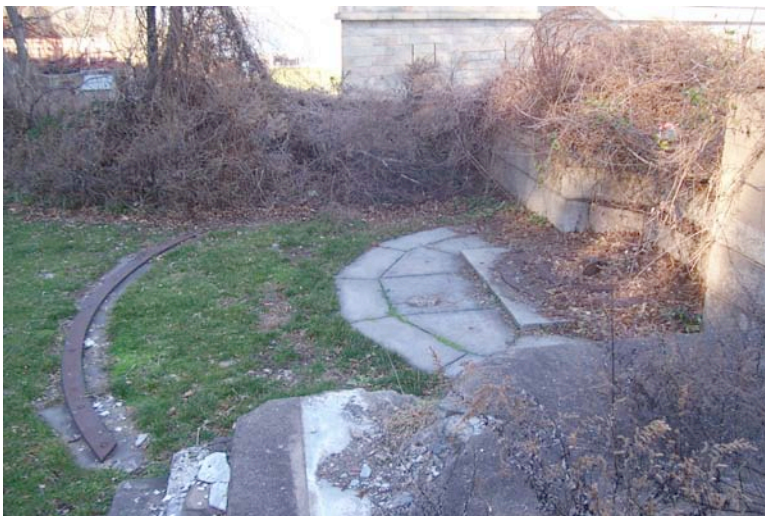
Figure 3.35: Although there is some cracking in the reinforced concrete platform of Battery Bacon, the concrete pad, iron pintel, and traverse circle remain in good condition. SUNY ESF, 2007.
