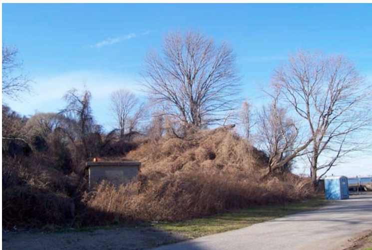
Figure 3.15: The southern end of Battery Catlin consists of a large earth mound measuring approximately 320 feet by 140 feet and rises to a height of forty-five feet above the level of the North Stone Dock SUNY ESF, 2007.
