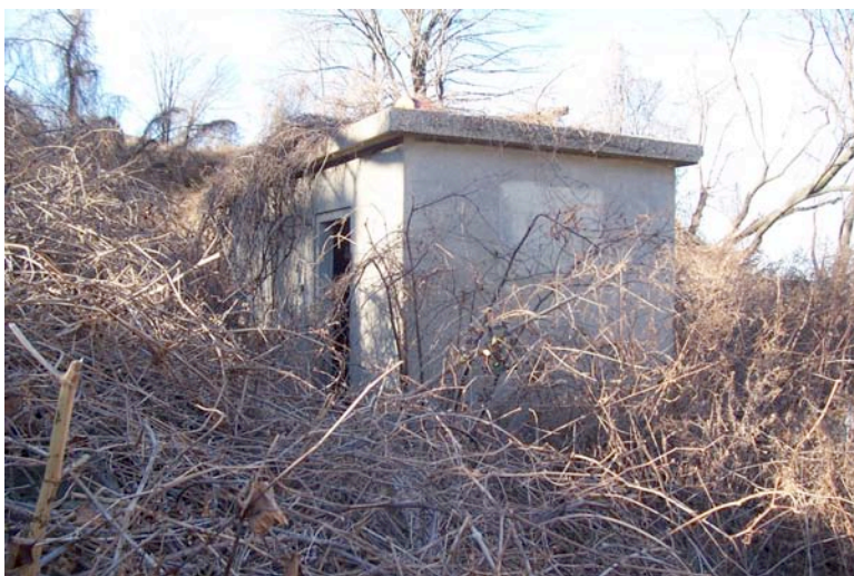
Figure 3.27: The small, one story, poured concrete shed on the west side of the dock road measures approximately 10 feet by 12 feet and has a concrete shed roof and a door opening on the southwest side. SUNY ESF, 2007.
