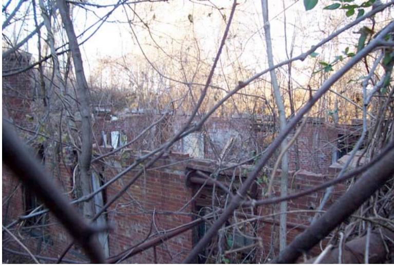
Figure 3.31: The Mine Casemate, measuring approximately sixty feet by seventy-five feet, is buried in the invasive and successional vegetation on Battery Catlin. The brick structure has window openings with slate sills, but has no roof. SUNY ESF, 2007.
