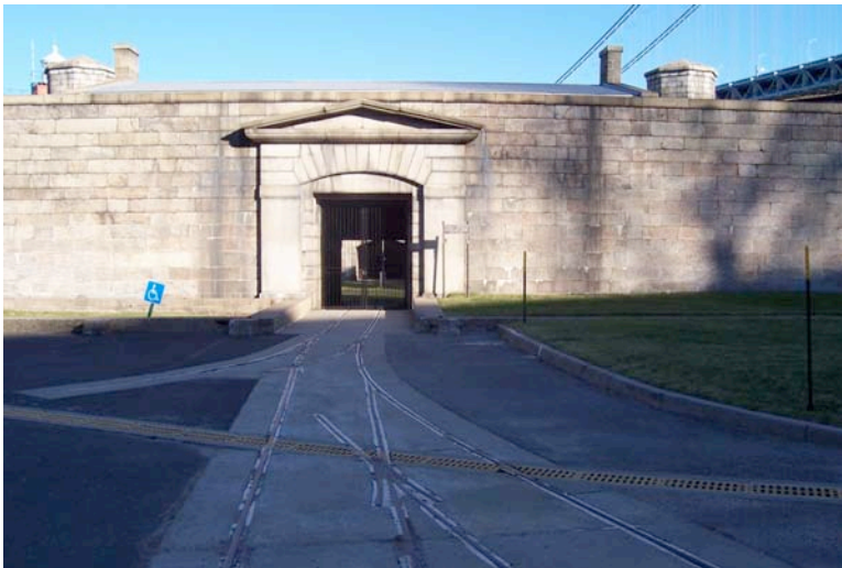
Figure 3.17: Surface Drain Inlet. SUNY ESF, 2007.
