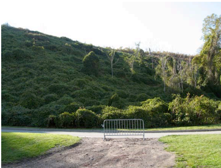
Figure 3.14: The engineered slope above Battery Weed exists in much the same configuration it had throughout the historic period. SUNY ESF, 2007.
