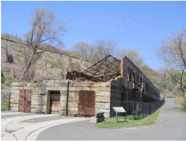
Figure 3.25: The torpedo storage building, a brick and stone structure with a steel truss, gable roof, measures approximately 230 feet by 40 feet. SUNY ESF, 2007.
