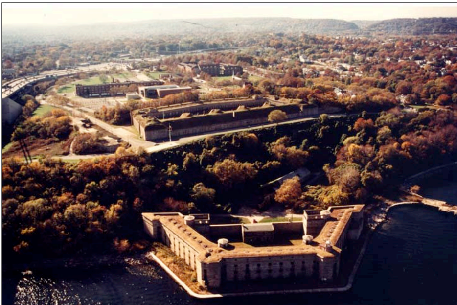
Figure 2.4: Aerial photograph looking west at the Fort Wadsworth military reservation with Battery Weed, the Overlook and Slope, and the North Stone Dock and Seawall in the foreground. Pier/Seawall Evaluation and Ferry Feasibility Study Fort Wadsworth, Staten Island, New York , Landgan Engineering and Environmental Services, 1995.
