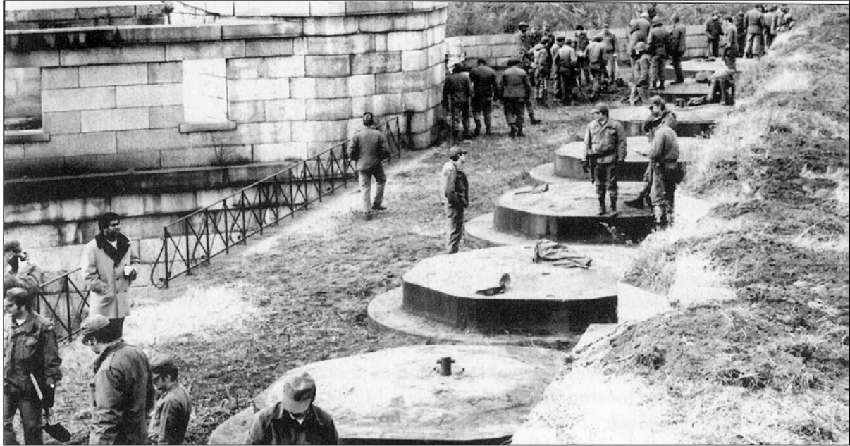
Figure 1.72: Photograph looking northwest from the parapet on the barbette tier of Battery Weed where an Army crew appears to be on a landscape maintenance detail, 1970. Gateway National Recreation Area Archives Photographic Collection.
