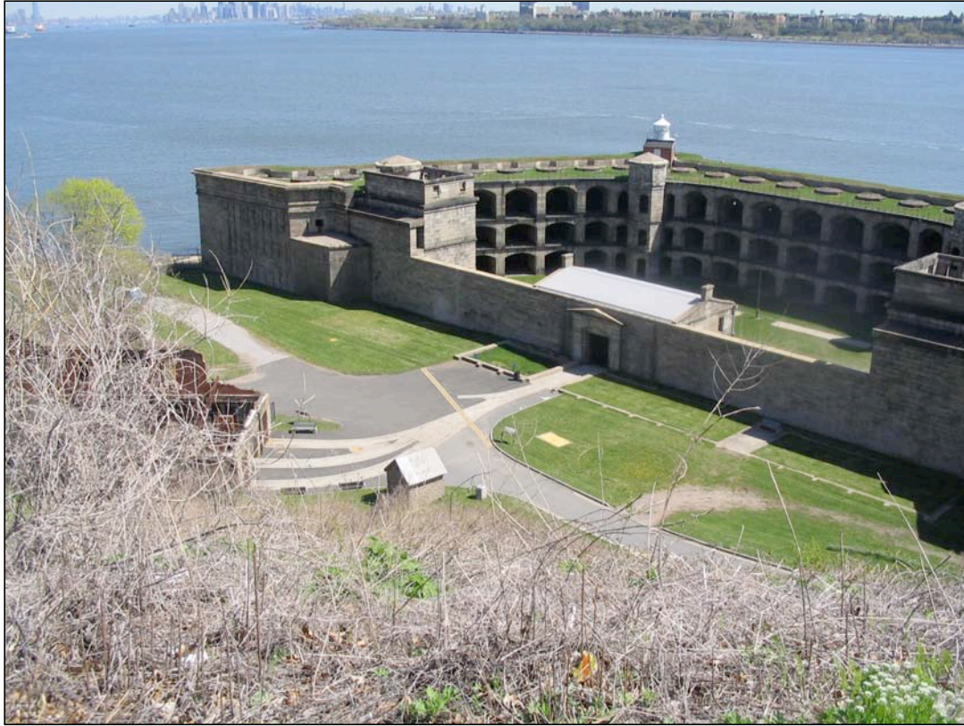
Figure 2.5: The Fortress Grounds looking northeast from the Overlook. SUNY ESF, 2007.
