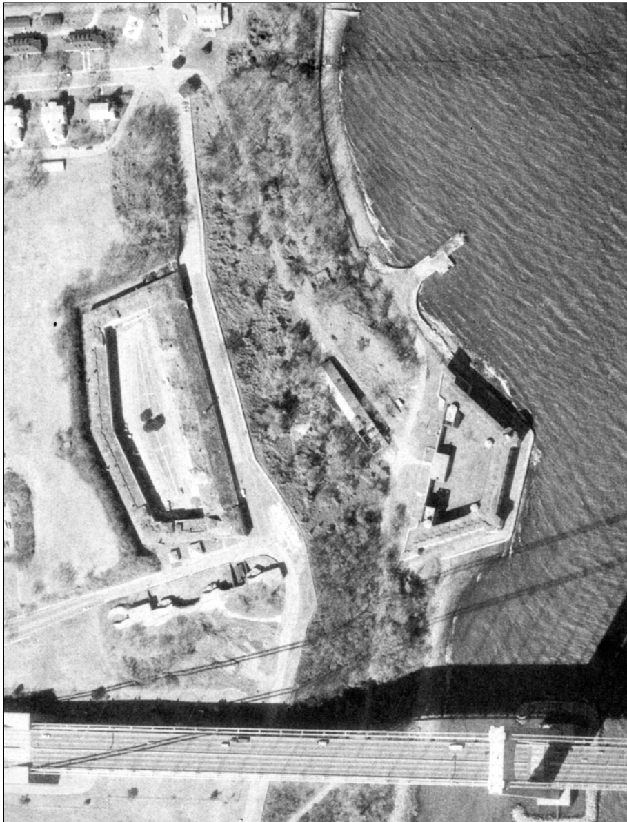
Figure 1.74: Satellite photograph showing Battery Weed, Fort Tompkins, the North Stone Dock, the Torpedo Storage Building and the Verrazano-Narrows Bridge at lower edge, 1990. Pier/Seawall Evaluation and Ferry Feasibility Study, Fort Wadsworth, Staten Island New York, prepared for the National Park Service, 1995, photograph by Aerial Viewpoint Houston, Texas.
