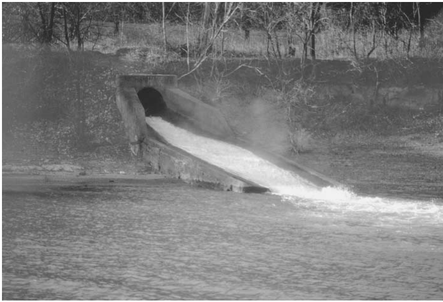
Figure 5: Combined sewer overflow, Allegheny River SOURCE: Author's photo.
