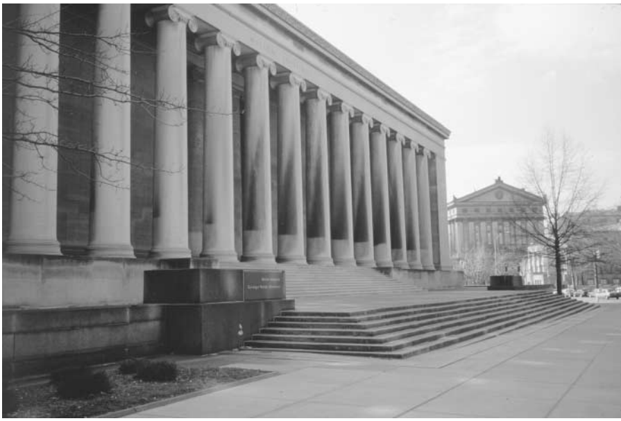
Figure 10: Building columns partially cleaned of soot, Mellon Institute of Science SOURCE: Author's photo.
