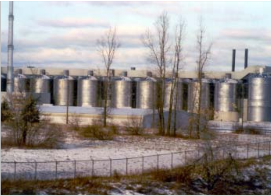
The proposed Northeast Biofuels site has several small fermentors already on site.
