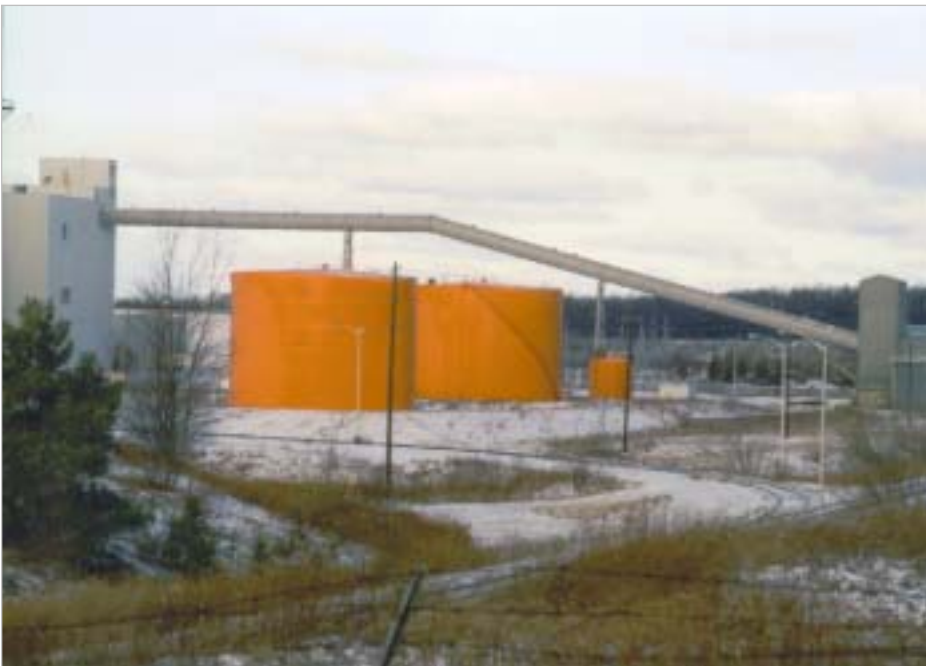
The former petroleum tanks at the proposed Northeast Biofuels site will be used for ethanol storage.
