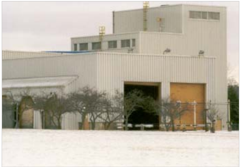
This building would be demolished in the renovation of the former brewery to make way for a new distillers grains drying and handling area.
