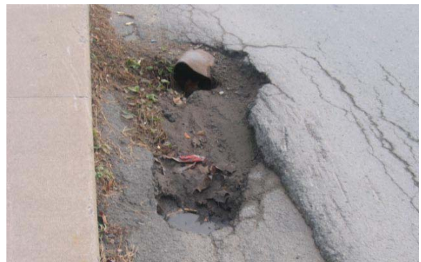
Figure 3. Pothole near back entrance to Rite Aid.
