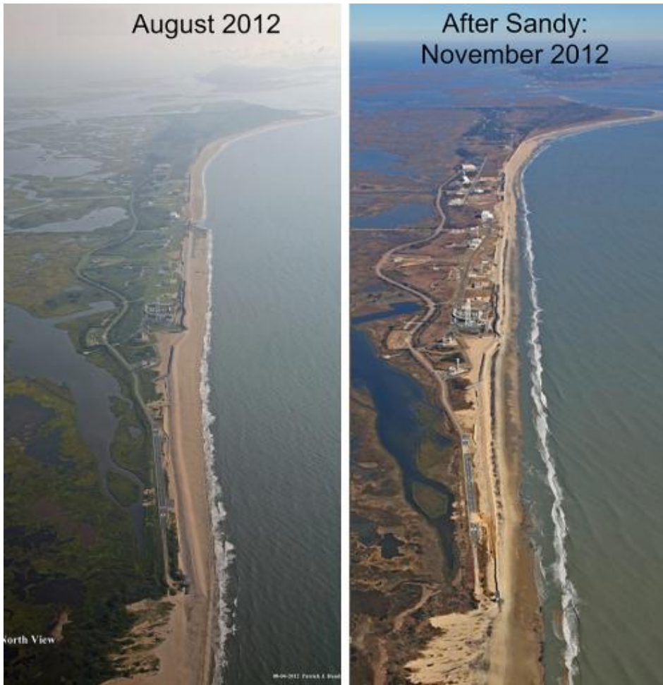
Aerial photographs of the NASA Wallops facility and coastline. On the left is from August 2012 after completion of a Shoreline Protection Project. On the right is from November 2012 after Hurricane Sandy swept by. Credit: NASA
