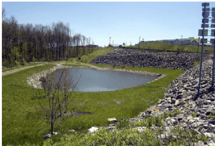
Wet Pond SMP at the Home Depot, Brewster, New York
