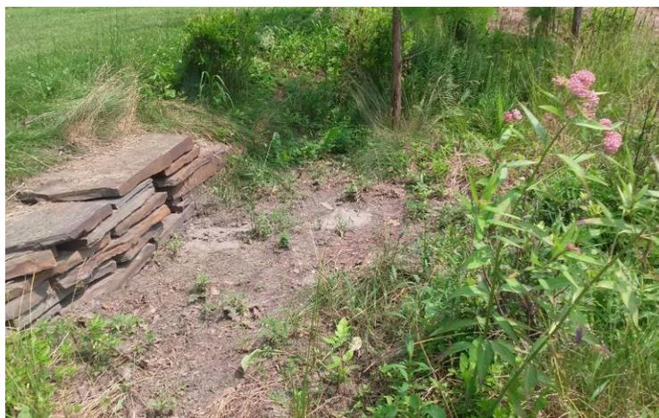
**Figure 7. Erosion surrounding inlet from Pass 2, resulting in poor vegetation vigor and survivability.**
