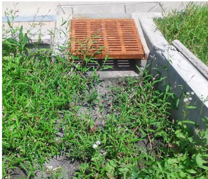
**Figure 5. Sediment build-up around the inlet of East Genesee, resulting in poor vegetation establishment and a compacted surface layer.**
