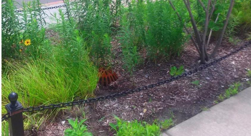
**Figure 4. Lack of sediment removal from South State resulting in homogenous topography and sediment build-up around site emergency overflow.**
