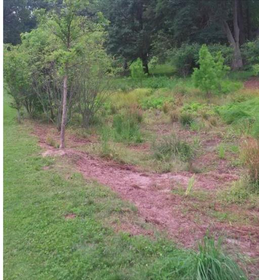
**Figure 8. Erosion on bank of Pass 2, resulting in poor vegetation vigor and survivability.**
