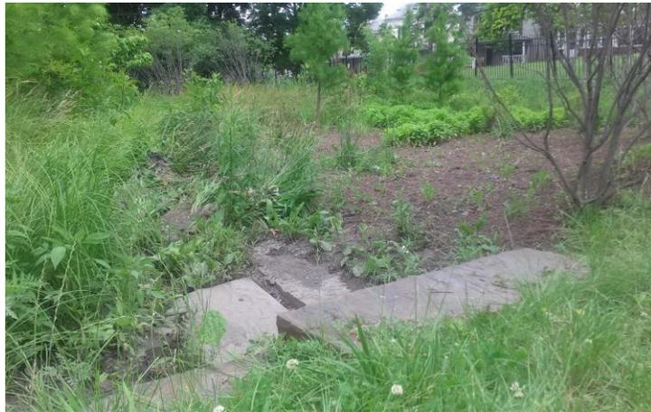
**Figure 6. Erosion and preferential surface flow path from inlet at Pass 1, resulting in poor vegetation vigor and survivability.**
