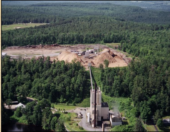
Combined Heat and Power
