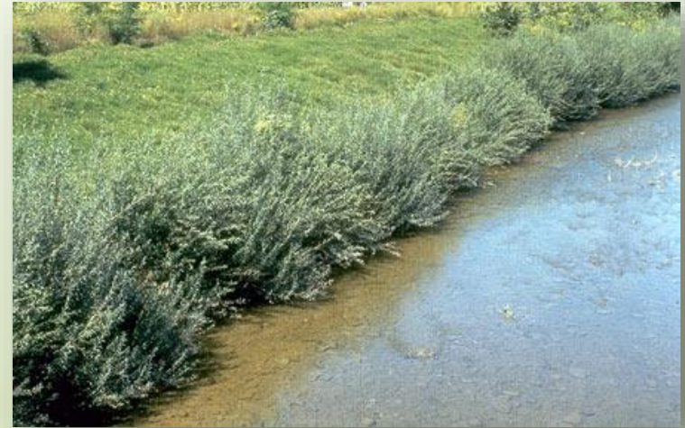
Stream Bank Stabilization
