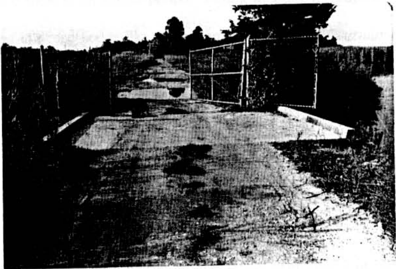
Fig. 3.7 - The concrete bridge is in excellent condition while the entry gate is in need of repair in order to make it more secure.
