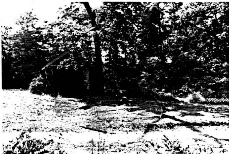
Fig. 3.34 - The stuccoed auto house has begun to lean due to the boggy soil on which it stands.
