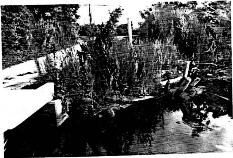
Fig. 3.6 - The entry road has begun to erode away due to the collapsed bulkheading.
