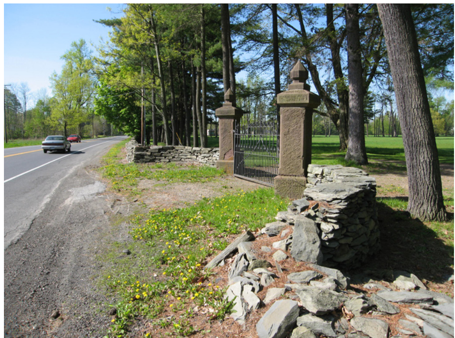
Figure 12: Recent view of the Home Road entrance looking south along the Post Road showing deteriorated condition of road shoulder, earthen roadbed, and stone wall. (SUNY ESF, 2007.)
