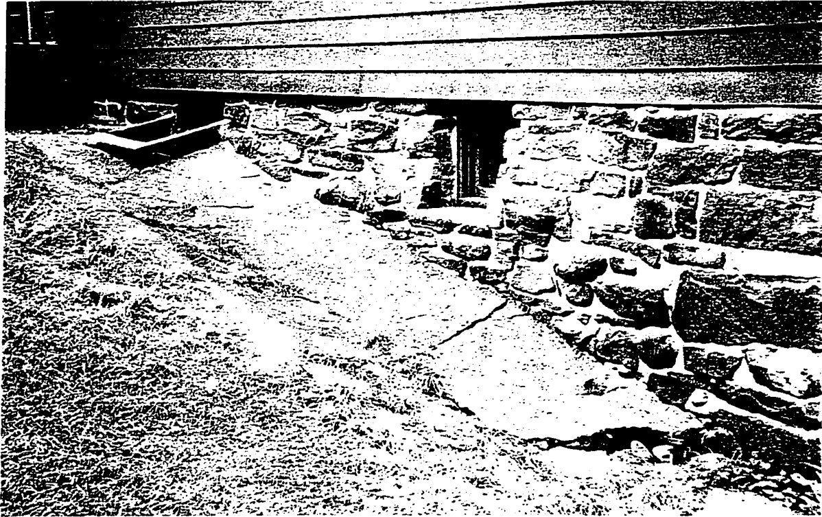
Figure 4.37: Concrete drainage gutter, looking northeast, 1997. (Photograph by the author).
