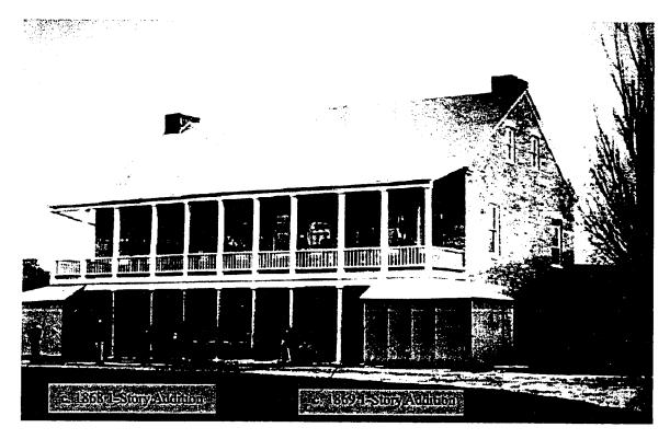
Fig. 3.29. "Enlisted Mens Barracks," looking southeast from Parade and showing c. 1868 and c. 1869 1-story additions, U.S. Army Signal Corps, 1870. Photograph courtesy of Fort Ontario State Historic Site. Annotated by R. Hetzler, SUNY ESF, 2002.
