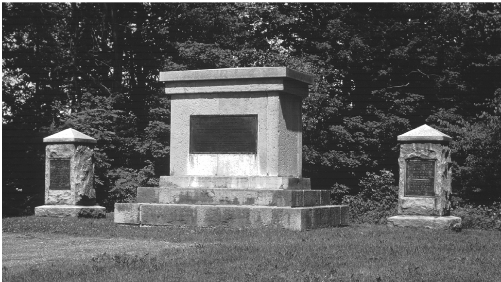
Figure 6.46: View northwest of Unknown Soldiers' Monument and relocated D.A.R. piers. Photograph by G. Curry, SUNY ESF, 1999.
