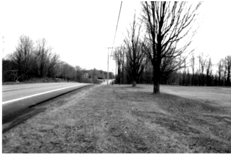
Figure 6.3: View west of the Road along east plateau illustrating pavement and drop in elevation across Battle Creek ravine. Photograph by J. Auwaerter, SUNY ESF, 1999.
