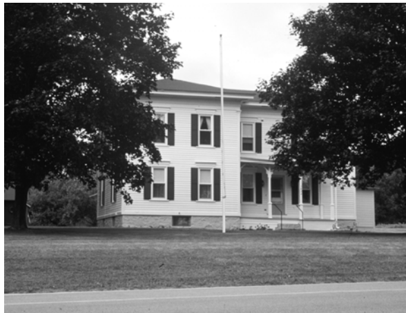
Figure 6.14: View south of former Ringrose farmhouse. Photograph by J. Auwaerter, SUNY ESF, 1999.
