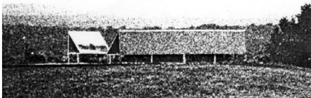
Figure 5.31: View north of panoramic photo-interpretive kiosk, c.1976. Detail of a photograph in Oriskany Battlefield files, Bureau of Historic Sites, Waterford.
