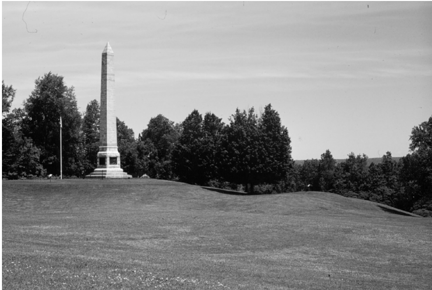
Figure 5.17: View northwest of the Battle Monument showing reforestation on the lowlands. Photograph by J. Auwaerter, SUNY ESF, 1999.
