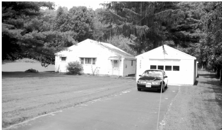
Figure 6.11: View north of Blair house. Photograph by J. Auwaerter, SUNY ESF, 2000. The Site is at the left beyond the white pine.
