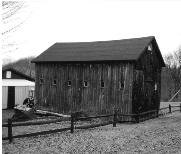
Figure 6.35: View northeast of the horse barn from the Road with maintenance garage at left. Photograph by J. Auwaerter, SUNY ESF, 1999.
