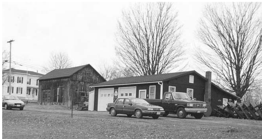
Figure 6.38: View southwest of the maintenance garage with horse barn and former Ringrose farmhouse to the right. The maintenance drive is in the foreground. Photograph by J. Auwaerter, SUNY ESF, 1999.
