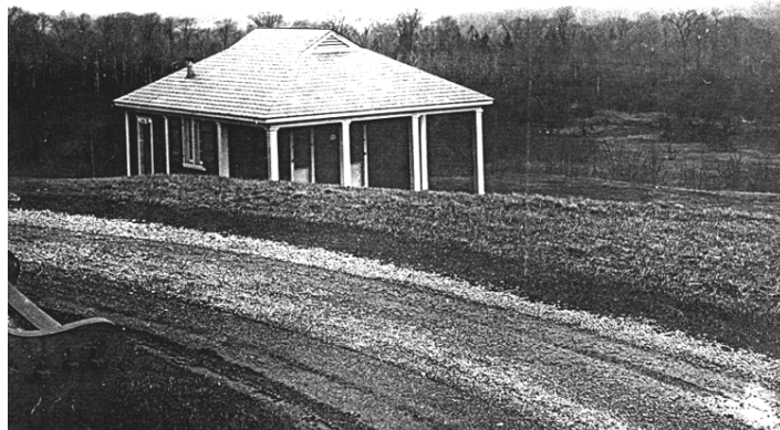
Figure 5.9: View northwest of the 1927 rest house with loop drive in foreground, c.1940. Oriskany Battlefield files, Bureau of Historic Sites, Waterford.
