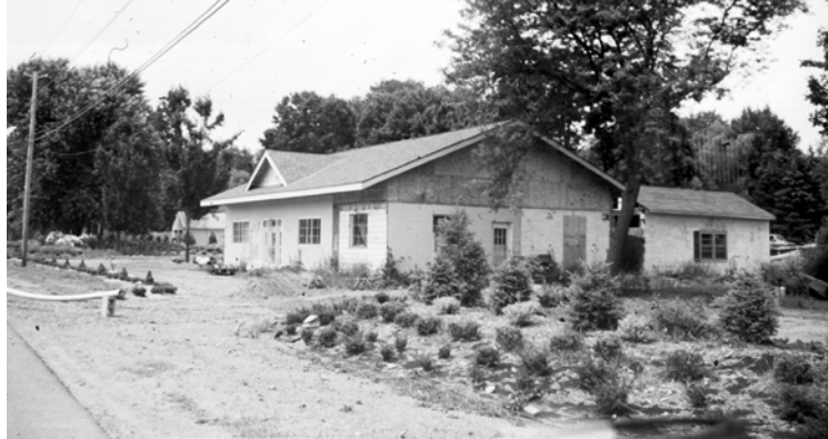
Figure 6.9: View northeast of Neidl building. Photograph by J. Auwaerter, SUNY ESF, 2000.
