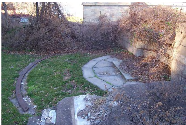
Figure 3.31: The gun emplacement (BS-9) at Battery Bacon (see T-3) built in c.1898 looking north showing concrete platform and parapet walls, iron pintle, and traverse circle. SUNY ESF, 2007.
