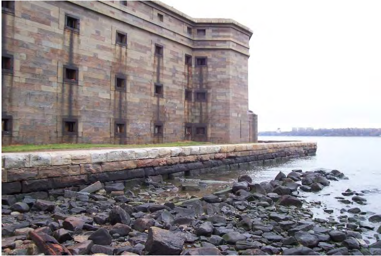
Figure 3.22: The seawall (BS-2) completed in c.1871, view looking northeast at section that forms the outer wall of the moat around Battery Weed. SUNY ESF, 2007.
