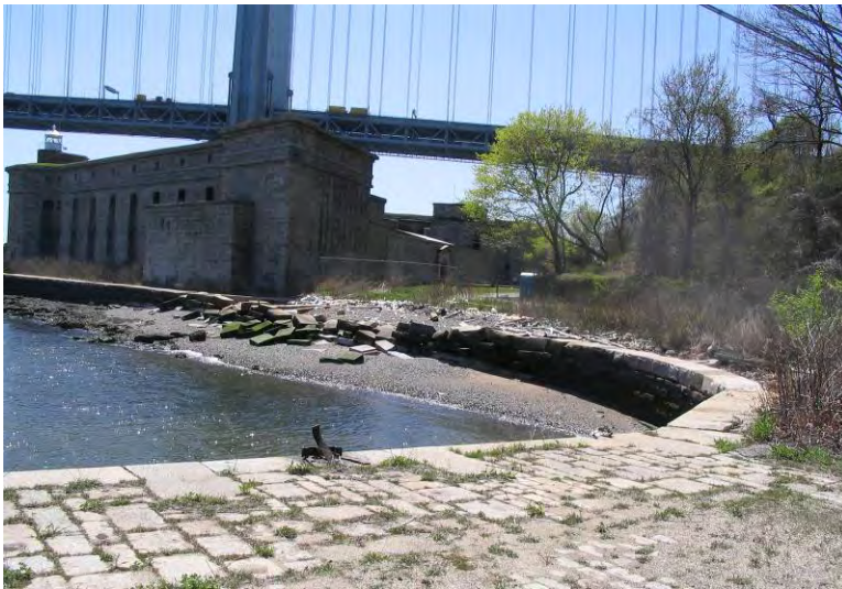
Figure 3.23: A section of the retaining wall section of the seawall (BS-2), looking south from the north dock showing a collapsed section. SUNY ESF, 2007.
