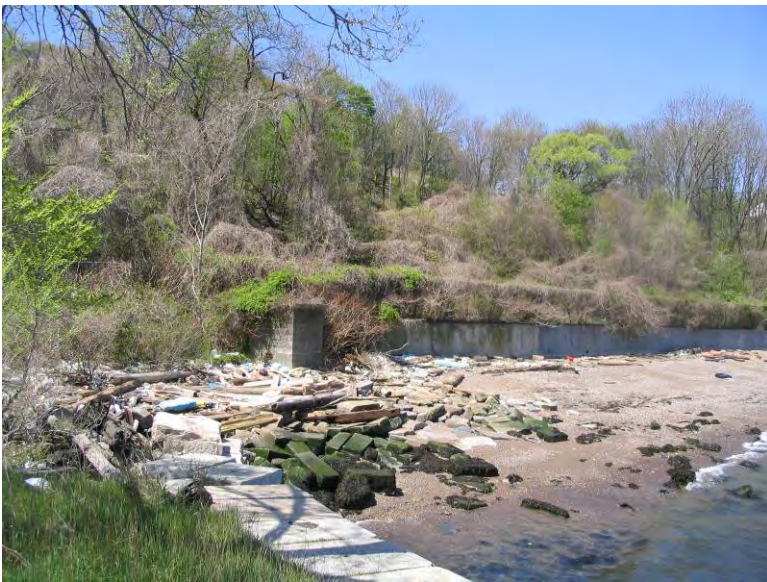
Figure 3.35: The partially vine-covered concrete seawall (BS-13) built in c.1938, view looking northwest with Battery Catlin in the background. In the foreground is a collapsed section of the granite seawall. SUNY ESF, 2007.
