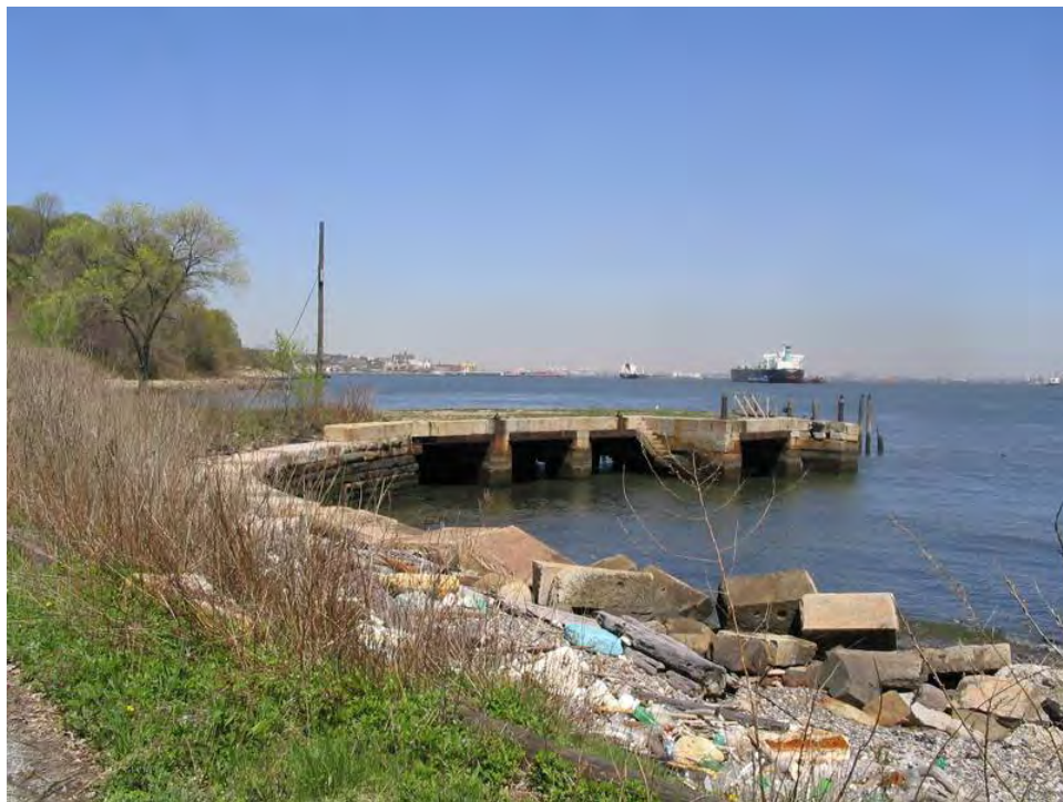
Figure 2.10: View looking north in 2007 showing the collapsed section of seawall and the north dock. The wood piles are remnants from a timber extension to the dock built in c.1907 and lost after 1960. SUNY ESF.
