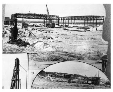
Figure 1.40: Collage of photographs showing construction of the trussed steel-frame hangars, c.1929. The bottom right photograph is looking south along Flatbush Avenue toward Barren Island (tree-covered area in background). (Photograph 18986, Gateway National Recreation Area Museum Collection.)
