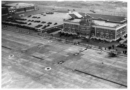
the same project, the WPA also installed four turn tables on the apron to either side of the tunnel hatches. These were installed in
