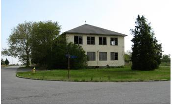
Figure 3.13: Near-historic (c.1949, top) and existing (2008) view of World War II-period temporary construction in the main barracks area. The photograph at the top illustrates the dispensary (87), the lower is a similar existing building, barracks 15 (72) showing current vacant condition and later siding. The plantings were added after 1945. (Top: Photograph 20302, Gateway National Recreation Area Museum Collection; bottom: SUNY ESF.)
