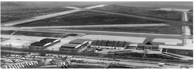
Figure 1.101: Looking east across Hangar Row showing the Air National Guard's nose hangar (265) built between the Administration Building and hangars 5-6 in 1965, from a later photograph, c.1992. In the rear is the apron that was enlarged by paving over turf between the taxiways most likely as part of the hangar construction. The World War II-era wing on the Administration Building was removed in c.1979. (Photograph 18888, Gateway **National Recreation Area Museum** Collection.)
