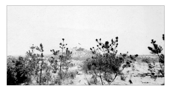
Figure 1.25. Casemated and earth covered Battery Harris, looking east, c.1942. The pine trees in the foreground, probably surrounding Battery Kessler, were planted to stabilize soils and/or camouflage the defensive works. (Gateway Museum Collection, GATE 1312)
