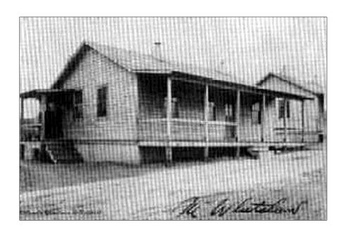
Figure 1.8. View of officer quarters, typical of the temporary frame construction built during World War I, c.1919. (National Archives).
