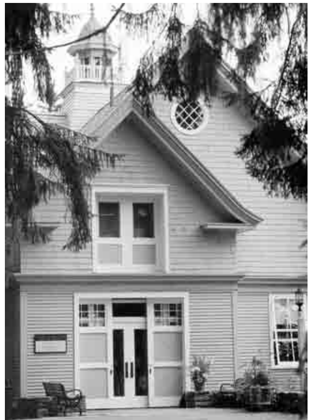
Figure 7.3: View of the front of the Carriage Barn following rehabilitation into a visitor center and park offices. Marsh-Billings-Rockefeller National Historical Park, 1999. In the foreground is the new stone-paved entranceway.
