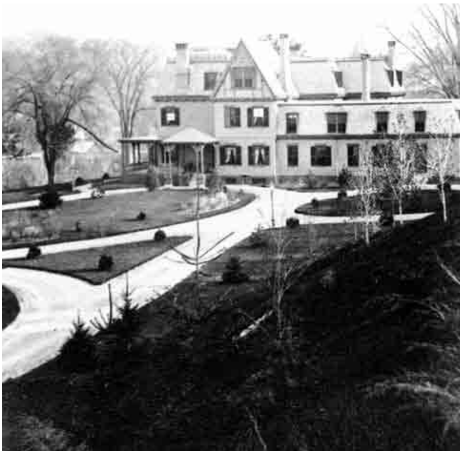
Figure 3.13: View of the north facade of the Mansion, c.1872. Billings Family Archives. The verandah and porte cochere are at the front (left) of the house, the one-and-a-half-story service wing is at the rear (right). Also visible are the gravel drives lined by cobblestone gutters and bordered by shrubs and herbaceous beds.
