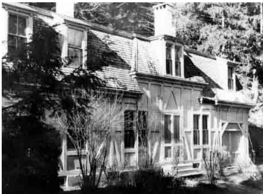
Figure 5.11: The front of the Laundry in its later years following removal of peaked roofs and other ornamental features, c.1945. Billings Family Archives. Note shrubs along the front, probably remnants of the 1902 Martha Brown landscape design.
