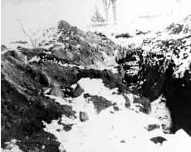
Figure 6.16: View east from the Mansion verandah in the winter of 1962, showing excavation undertaken for construction of the Mansion fallout shelter. Courtesy Mimi Bergstrom, Woodstock, Vermont.
