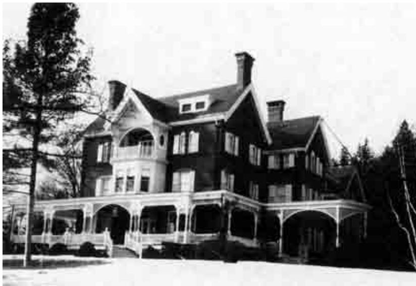
Figure 6.21: View of the front and north side of the Mansion, showing one of the newly planted white pines in the lawn, December 1967. Assessment Records, Town of Woodstock.
