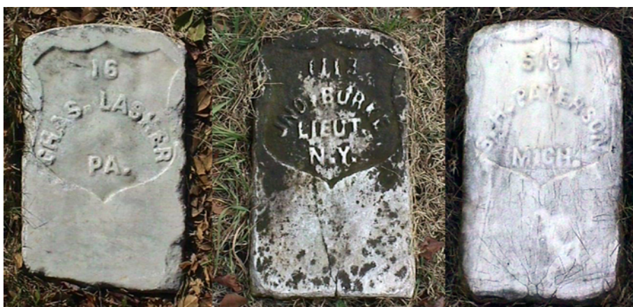
Figure 2.29: Representative first-generation recessed-shield headstones installed in 1877 and transformed into flat markers in 1934. These photographs illustrate characteristic chipping, cracking, weathering, and staining. The bases were cut or broken off. (Petersburg National Battlefield, 2005.)
