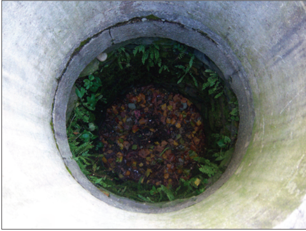
Figure 2.38. The interior of the spring well showing the existing water level (leaf-covered) and lower fern-lined stone walls that predate the courtyard. The upper limestone section was added in c.1933. (Roger Williams National Memorial, 2009.)
