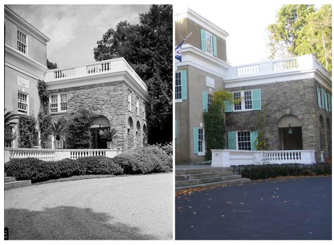
Figure 8: Comparison of paving character showing gravel-surfaced turn-around in July 1941 and the existing black asphalt that replaced it. These images also changes to the foundation shrubs. (Left: Digital image 115847pr, Historic American Building Survey, Library of Congress American Memory Collection; right: SUNY ESF, 2005.)
