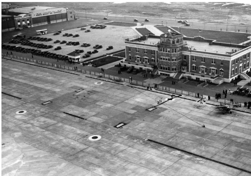
Figure 1.58: View of the gate area and apron looking southwest showing recently built rectangular passenger tunnel hatches and rotating platforms, c. 1936. The annotations are on the original photograph. The hipped-roof booth at the corner of the parking lot was probably removed with opening of the Field House in 1937. (Photograph 22017, Gateway National Recreation Area Museum Collection.)
