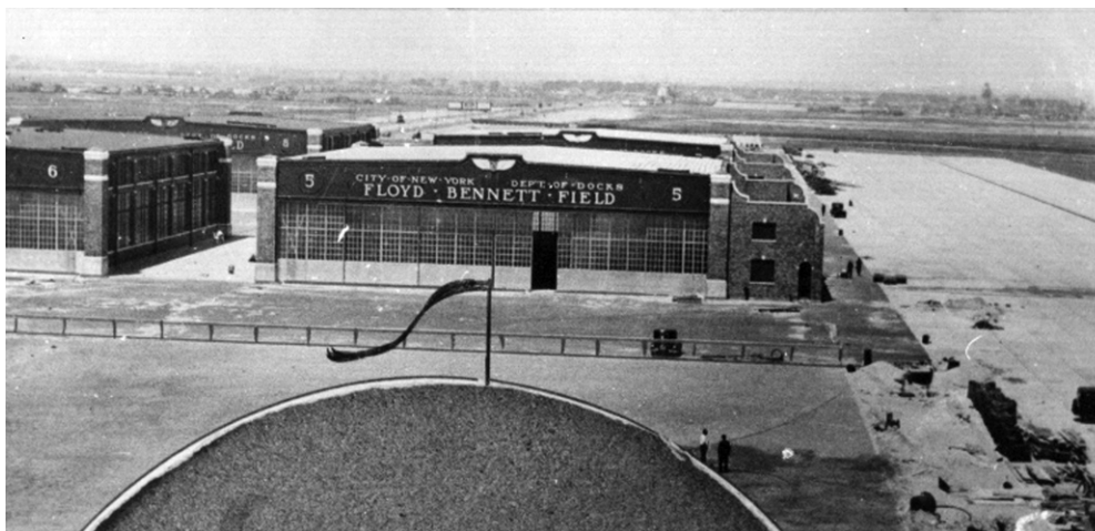
Figure 1.41: Hangars 5-8 looking north with the concrete apron at right and Flatbush Avenue at left, c.1930. The wings on the outer sides of the hangars are the lean-tos, and the dark ground surfaces are asphalt pavers. (Photograph 18883, Gateway National Recreation Area Museum Collection.)
