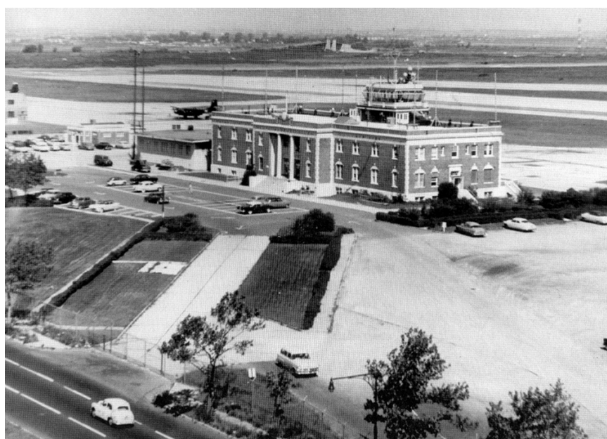
Figure 1.75: View of the airport entrance area looking northeast showing cyclone fence closing off entrance drives and frame addition to the Administration Building (at left), from later photograph c.1954. Also visible is the replacement control tower cab and remaining hedges and shrubs. (City of New York municipal archives, reproduced from Judith A Quinn, "Historic Structures Report, The Administration Building," 2004.)
