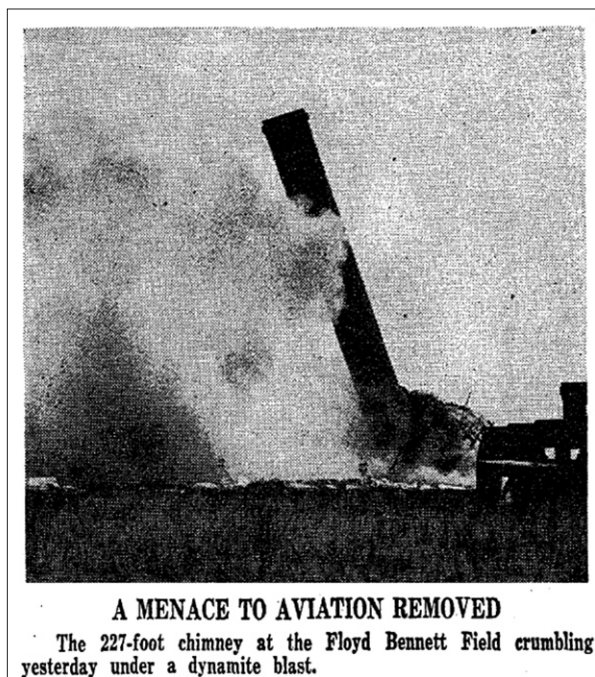
Figure 1.61: Photograph of the New York Sanitary Utilization Company chimney being demolished to clear the flight path of runway 12-30. ( New York Times , 21 March 1937. Copyright New York Times.)
