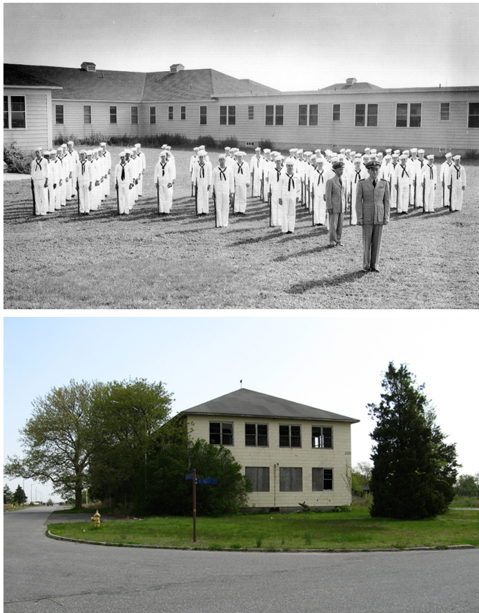
Figure 3.13: Near-historic (c.1949, top) and existing (2008) view of World War II-period temporary construction in the main barracks area. The photograph at the top illustrates the dispensary (87), the lower is a similar existing building, barracks 15 (72) showing current vacant condition and later siding. The plantings were added after 1945. (Top: Photograph 20302, Gateway National Recreation Area Museum Collection; bottom: SUNY ESF.)
