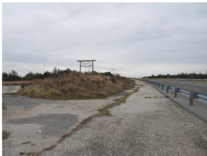
Figure 2.17 (top): View north along the four-lane entrance road constructed over runway 15-33 (taxiway 10), May 2008. Note original concrete pavement of the runway visible to the right of the guiderail. (SUNY ESF.)
