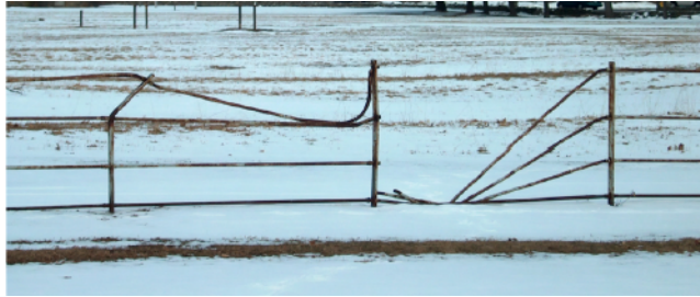
New damage to the steel pipe fence.
