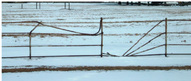
New damage to the steel pipe fence.
