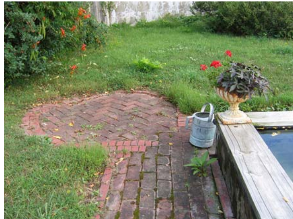
Fig. 28 2007 Pool Garden northeastern herringbone pattern paving detail
