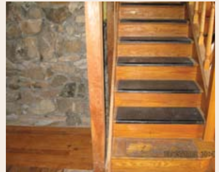
Before: Filled-in fireplace stones hidden behind former closet.
