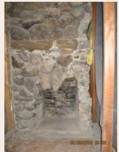
During: The cemented rubble has been removed.
