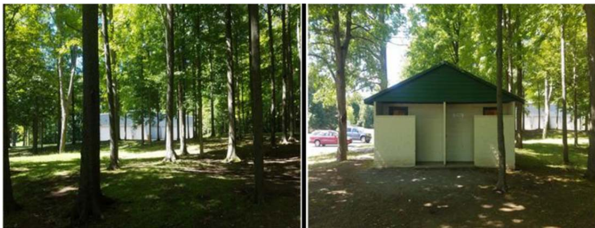
Figure 2. Parks and recreation building (left). Restroom/storage building (right)
