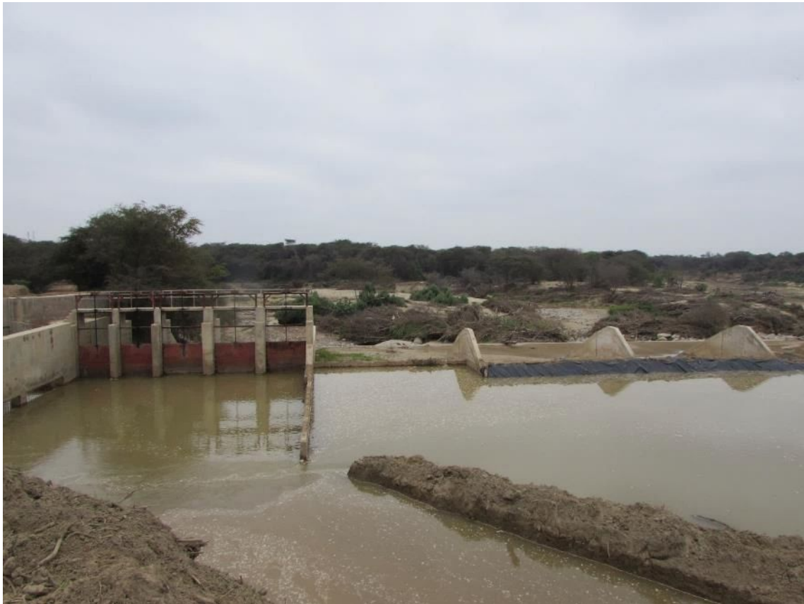
Figure 10: Diversion dam at Pómac Forest, looking west. Water passes to the canal through control gates (left) while the La Leche River flows over a concrete embankment (right). Note the tamarisk grouping in the center of the photograph.
