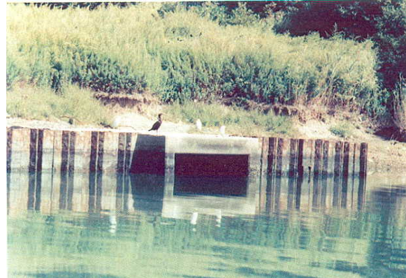
Storm sewer outfall in Fresh Creek Photograph: L. Kachalsky, O'Brien & Gere
