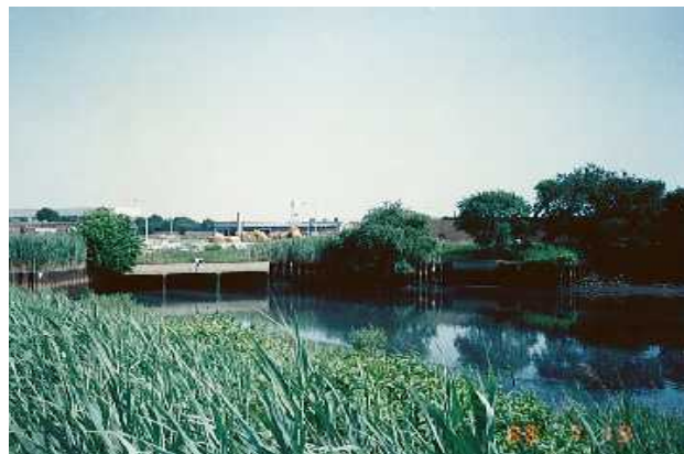
CSO outfall at Bergen Basin. Photo: L. Kachalsky, O'Brien & Gere
