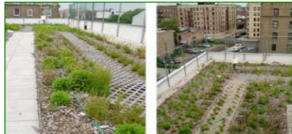
One of Gaia Institute's green roof projects in the New York City area; Source: Gaia Institute
