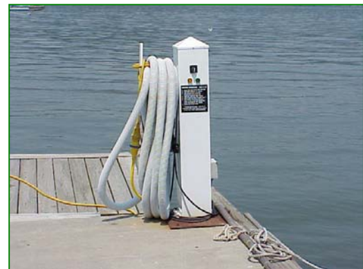
Paerdegat Basin Pump-Out. Source: NYCDEP
