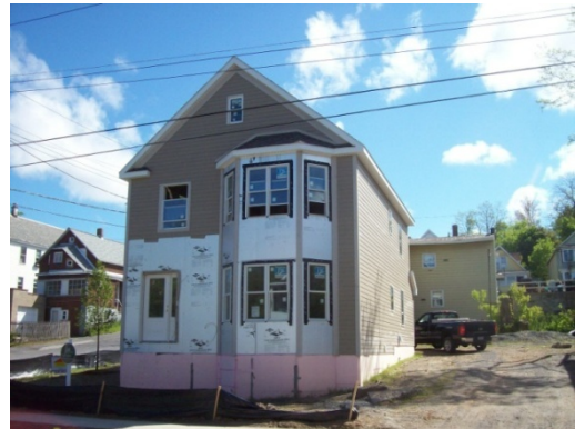
The City of Schenectady is sponsoring construction of affordable, highly efficient homes to replace deteriorating buildings.
