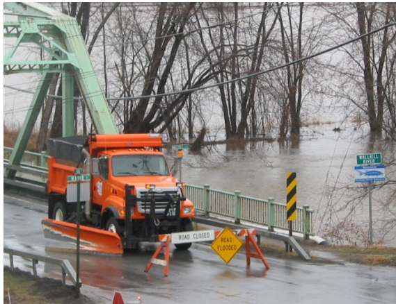
Transportation may be disrupted more often and more severely as heavier rains flood roads and bridges located near New York's many rivers and streams.
