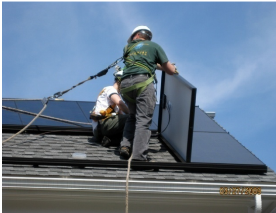
Solar panels on the Town Hall roof in the Climate Smart Community of Red Hook are reducing power bills so successfully that the town has applied to expand the installation and develop renewable energy improvement projects for other local government facilities. (Photo courtesy of Town of Red Hook)
