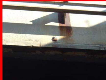
If the hooks are broken, bent or missing, fix or replace them
