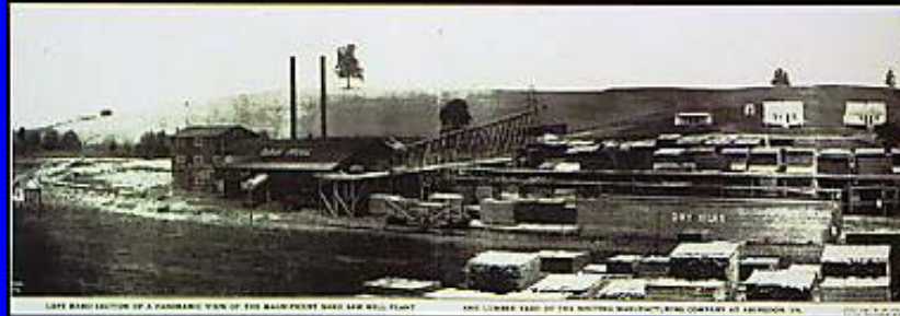
LEFT: EARLY SECTION OF A PIONEER YARD OF THE BIRD-PHANT SAW MILL, FLAHO. AND LIBBYE 1880: IN THE NORTH-WESTERN, KING COMPANY AT BIRCHMOUNT, WA.
