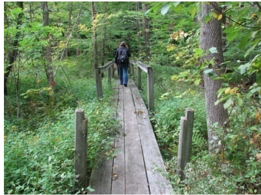
Figure 8. Footbridge allowing travel over marshy area east of recently remodeled lodge.
