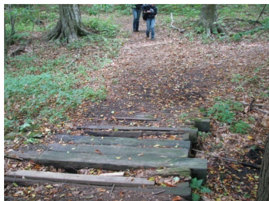
Figure 9. Second footbridge allowing travel over wet areas.
