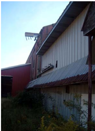
West side of the building complex
