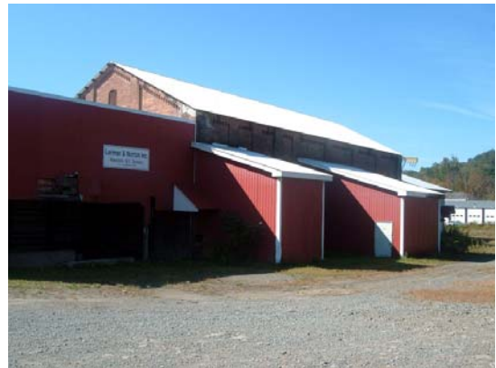
View of the front of the building.
