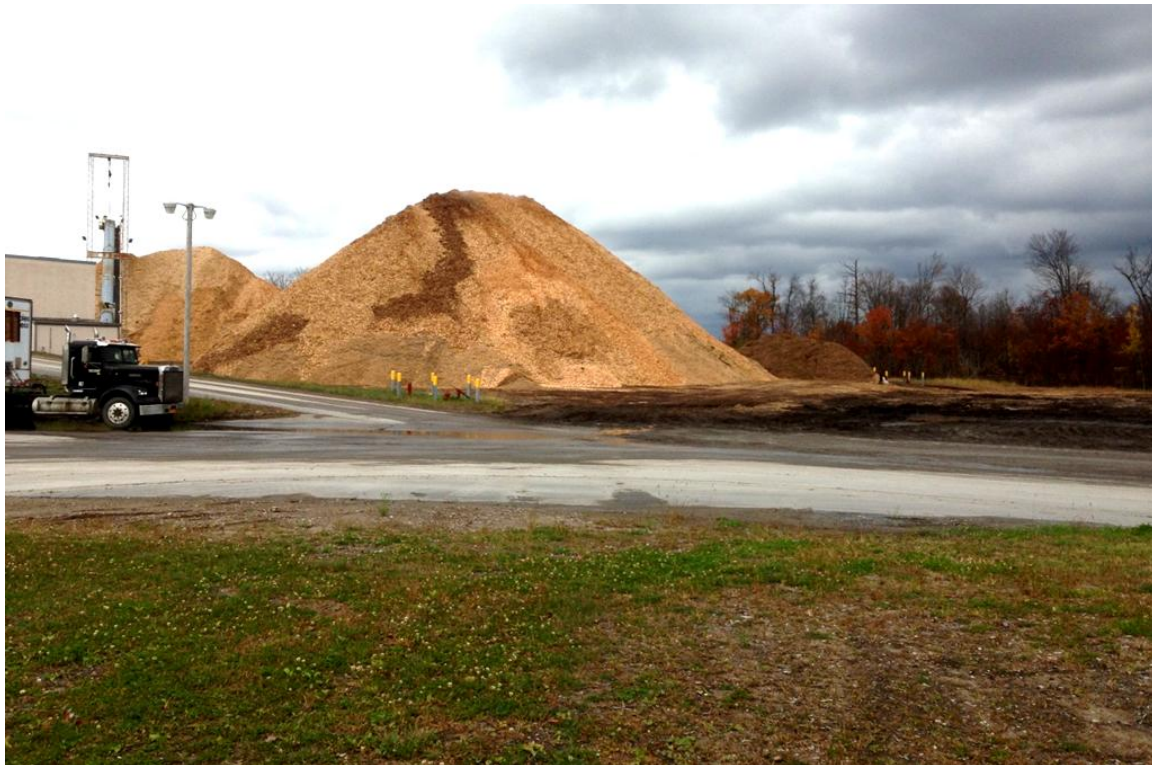
Image 14: Chip storage at ReEnergy Lyonsdale biopower facility showing forest wood chips (foreground) and shrub willow chips harvested in fall 2013 in background
