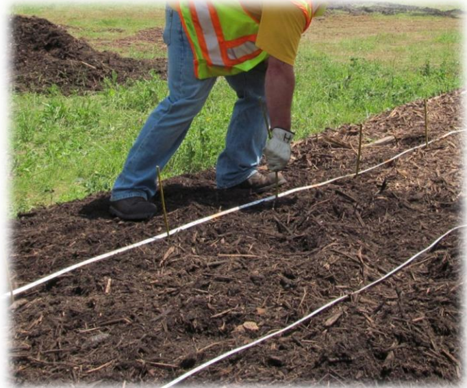
Figure 5 (left) – Applying wood mulch to a planted shrub-willow snow fence Figure 6 (right) – Planting cuttings directly through mulch and landscape fabric underneath Photos by SUNY ESF
