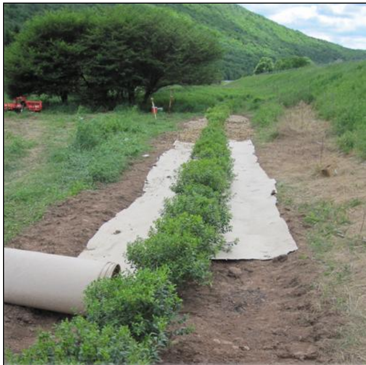
Paper-based landscape cloth used with plants intended to control near snow.
