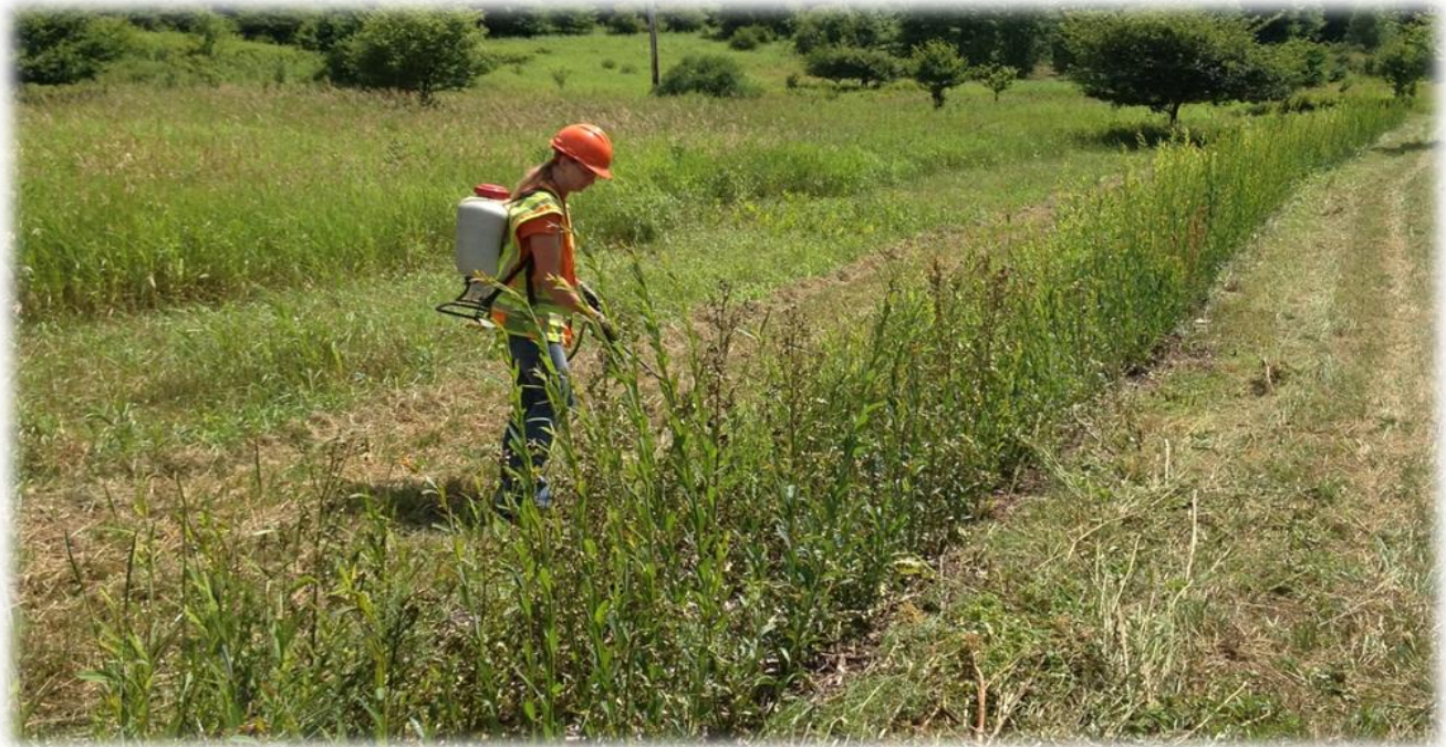
Figure 1- Maintaining 8+ feet wide mowed strips on either side of the fence, and regularly applying deer repellent to the fence were effective weed and browse controls on this 1 year old shrub-willow snow fence on Route 10 in Beerston, NY. Photo by SUNY ESF
