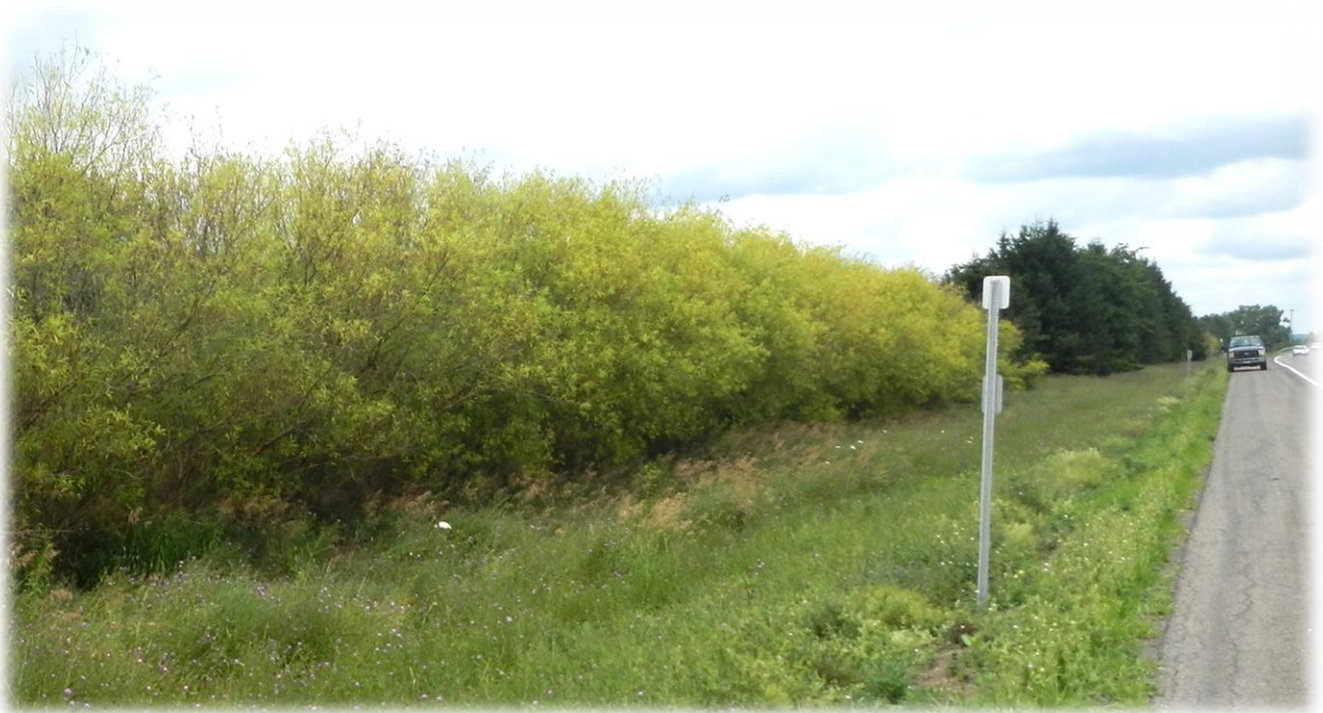
Figure 42: Living snow fence Preble-A-willow-9 from the edge of I-81 SB in late summer 2012
