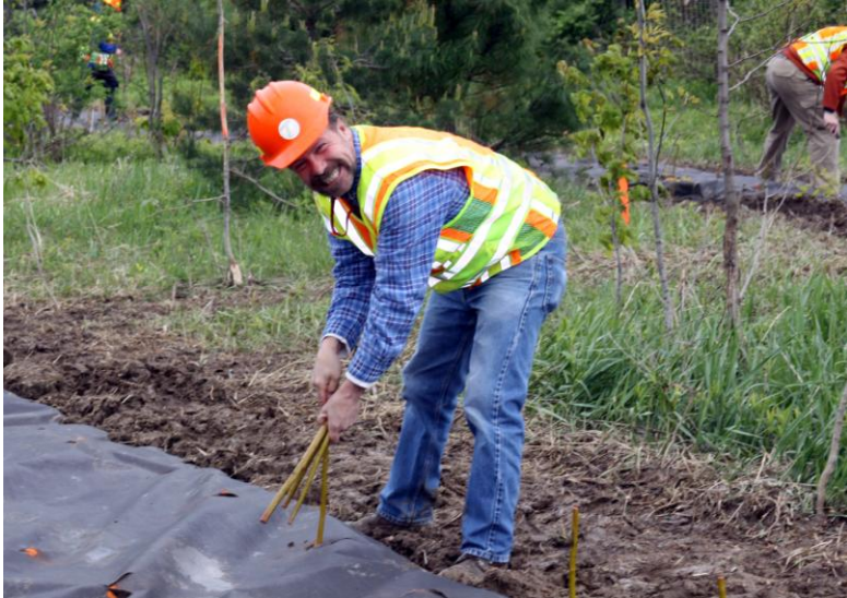
Left and right pictures: depending on the soil, willows may be placed with a mallet or by hand. In the left picture, Tim Volk installs with a mallet; in the right, John Harvey and an unidentified NYSDOT employee install willows by hand.
