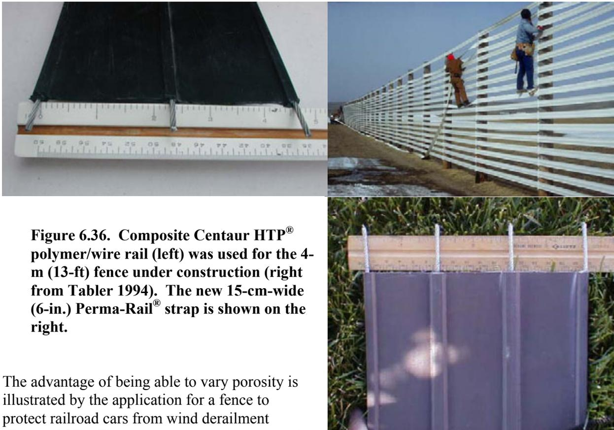
**Figure 6.36. Composite Centaur HTP<sup>®</sup> polymer/wire rail (left) was used for the 4-m (13-ft) fence under construction (right from Tabler 1994). The new 15-cm-wide (6-in.) Perma-Rail<sup>®</sup> strap is shown on the right.**
