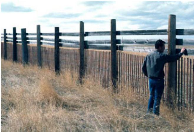
**Figure 6.27. Combination of lath fencing and horizontal boards.**
