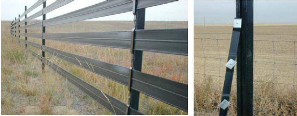
**Figure 6.41. "C" channel post with adjustable brackets.**
