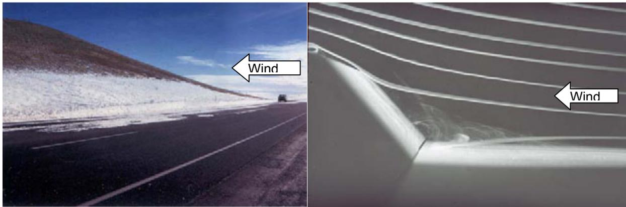
**Figure 8.19. Upwind drift in cut sections is caused by flow divergence as wind approaches a downwind obstacle. View on right is a wind tunnel smoke simulation, photo courtesy of the University of Wyoming.**
