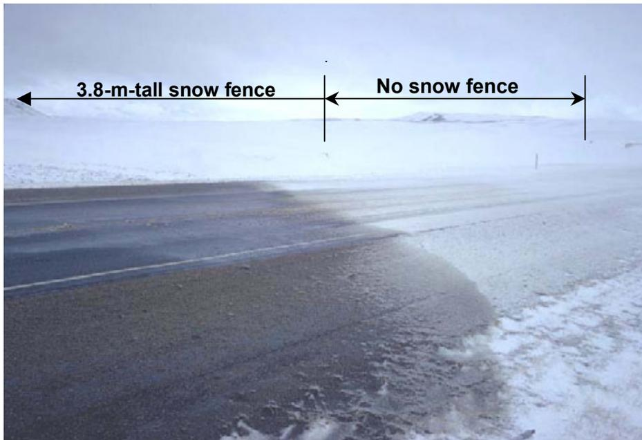
**Figure 2.11.** This transition from frozen slush to wet pavement corresponds to the beginning of the area protected by a 3.8-m-tall (12.4-ft) snow fence located about 150 m (500 ft) upwind. The upper corner of the fence, which extends to the left but is hidden behind the drift, is visible near the center of the picture. The area on the right side of the transition is unfenced (Mile 247.6, Wyoming I-80). (From Tabler and Furnish 1982).
