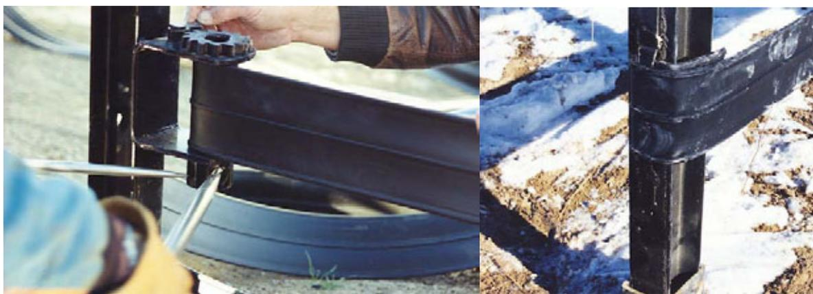
**Figure 6.38. Left: Ratchet winch permanently attached to end of fence line facilitates installation and maintenance. Right: Method of attaching "dead" end to post.**
