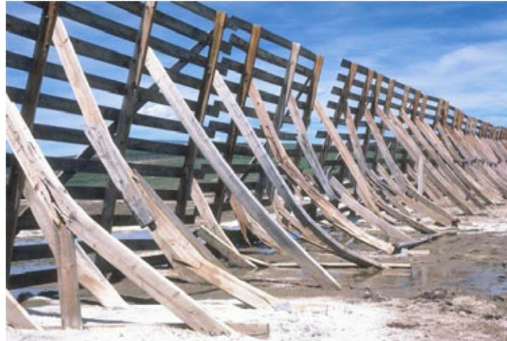
Lumber for the Wyoming fence can be purchased precut, predrilled, and treated with wood preservative.
