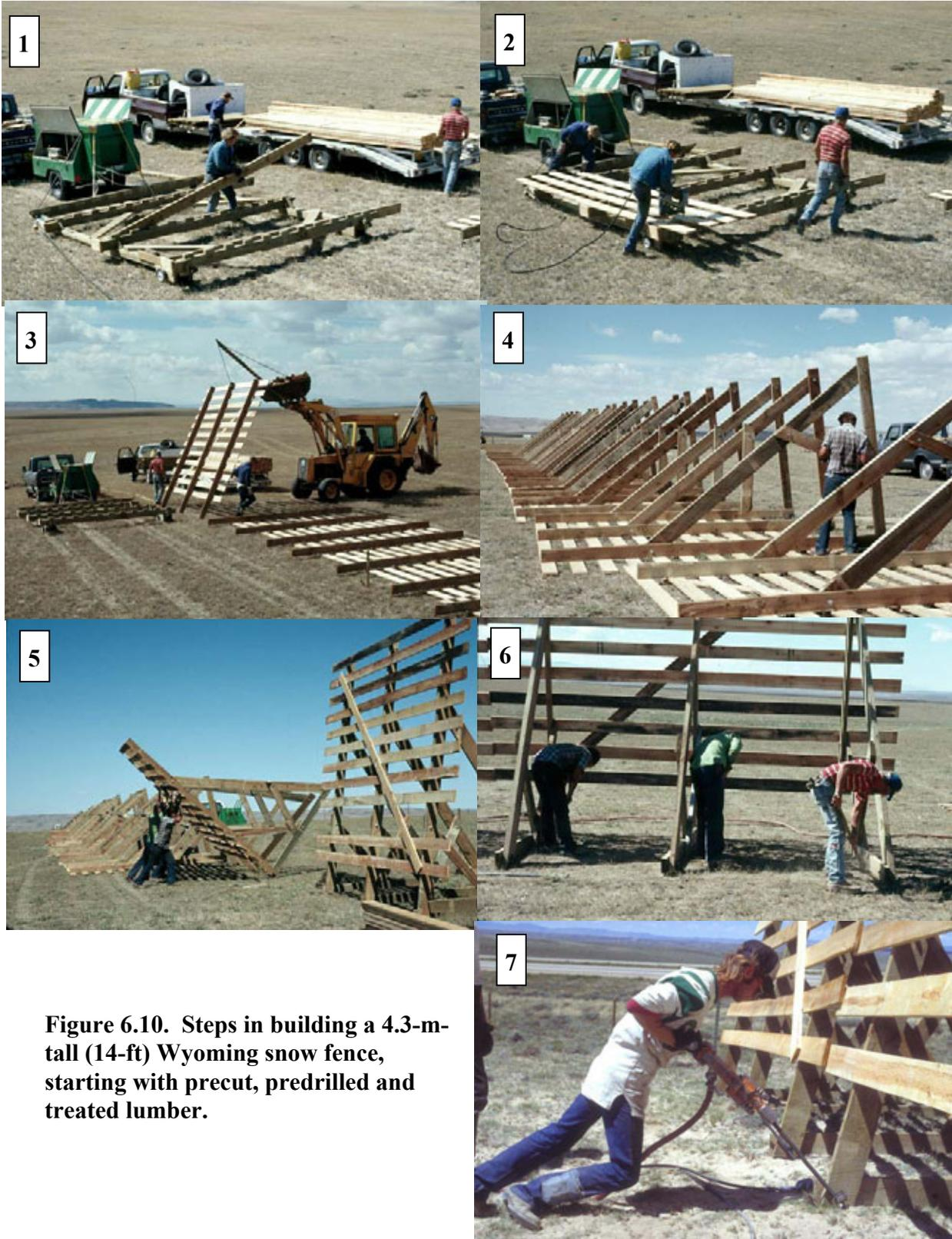
**Figure 6.10. Steps in building a 4.3-m-tall (14-ft) Wyoming snow fence, starting with precut, predrilled and treated lumber.**
