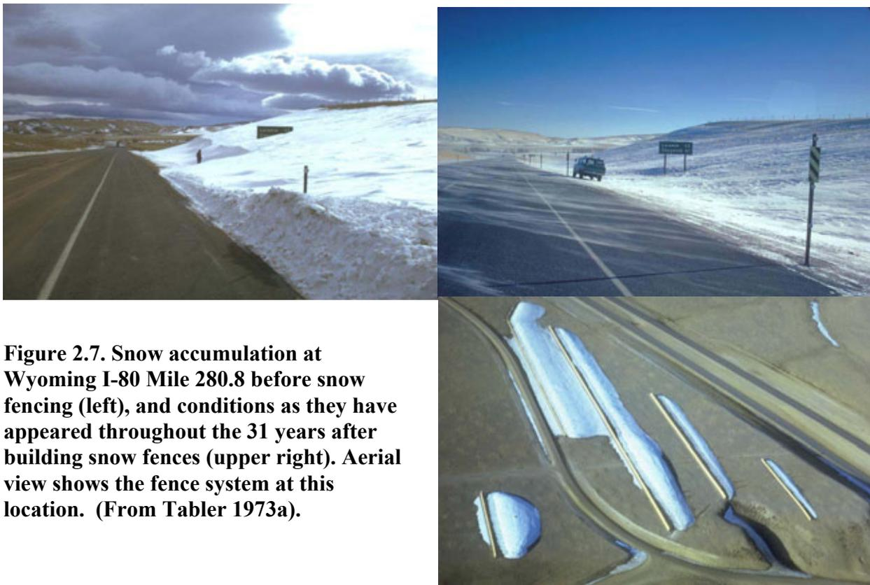
**Figure 2.7. Snow accumulation at Wyoming I-80 Mile 280.8 before snow fencing (left), and conditions as they have appeared throughout the 31 years after building snow fences (upper right). Aerial view shows the fence system at this location. (From Tabler 1973a).**
