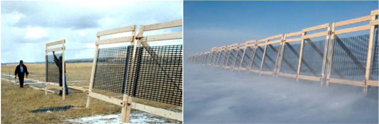
**Figure 6.53. The 2.0- and 2.4-m-tall (6.5- and 8-ft) patented portable fence design uses a wooden framework to support the Tensar<sup>®</sup> fencing material (left from Tabler 1994). The 2.4-m version is shown in these views.**
