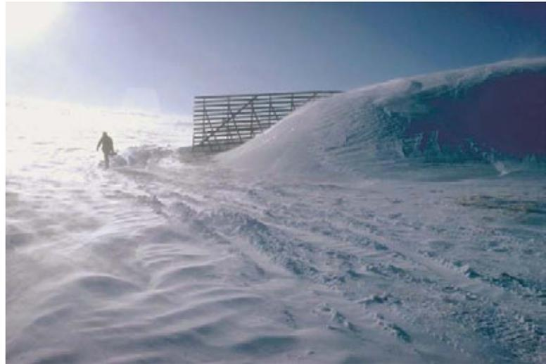
**Figure 3.43. Extent of the three-dimensional rounding of drift ends that constitutes the end effect (Tabler 1986).**
