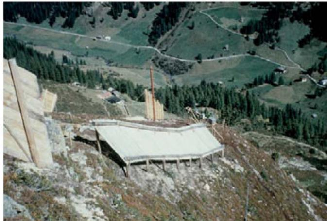
In Japan, very large jet roofs have been used to reduce snow deposition in road cuts, and constitute one example of blower fences, or *yudō-saku*. Large blower fences designed to reduce snow accumulation in road cuts (Figures 6.63 and 6.64) can be effective in reducing snow deposition. Although collector fences can be much more efficient, the value and agricultural use of land in Japan has resulted in the preferential use of blower fences placed close to the road.
