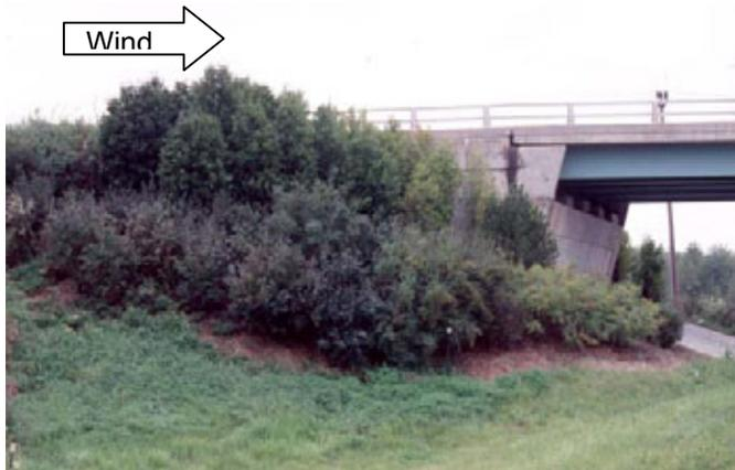
**Figure 7.23. This planting was reported to be successful in reducing drifts at this grade separation.**
