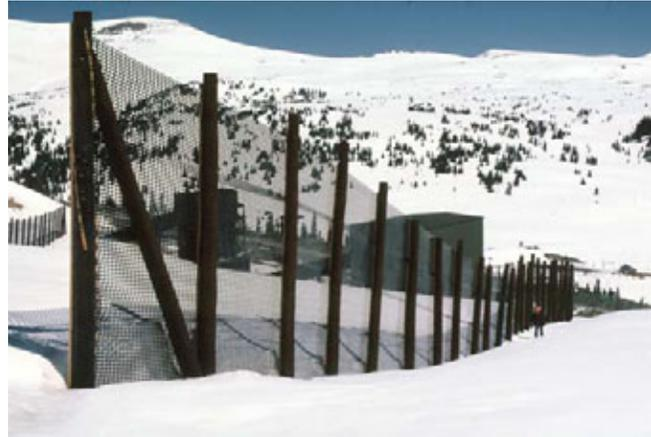
The preceding guidelines were developed when plastic netting was the only synthetic material available for fences. Now that the composite materials described in sections 6.3.7.3.4 and 6.3.7.3.5 are available, plastic netting is no longer recommended for permanent fences taller than 1.8 m (6 ft) or so.
