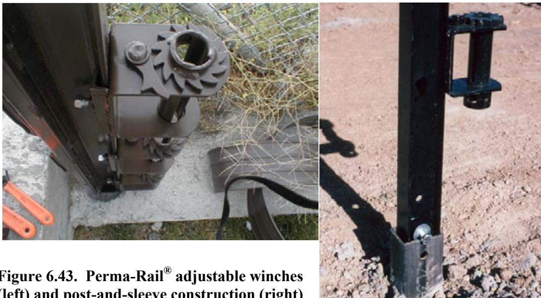
**Figure 6.43. Perma-Rail<sup>®</sup> adjustable winches (left) and post-and-sleeve construction (right) allow adjustment of bottom gap in uneven terrain. Photo left courtesy Perma-Rail International.**
