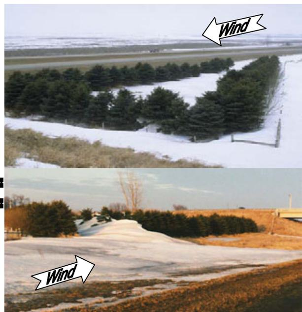
**Figure 7.22. A combination of trees and shrubs can reduce blowing snow problems at grade separations (Tabler 1994).**
