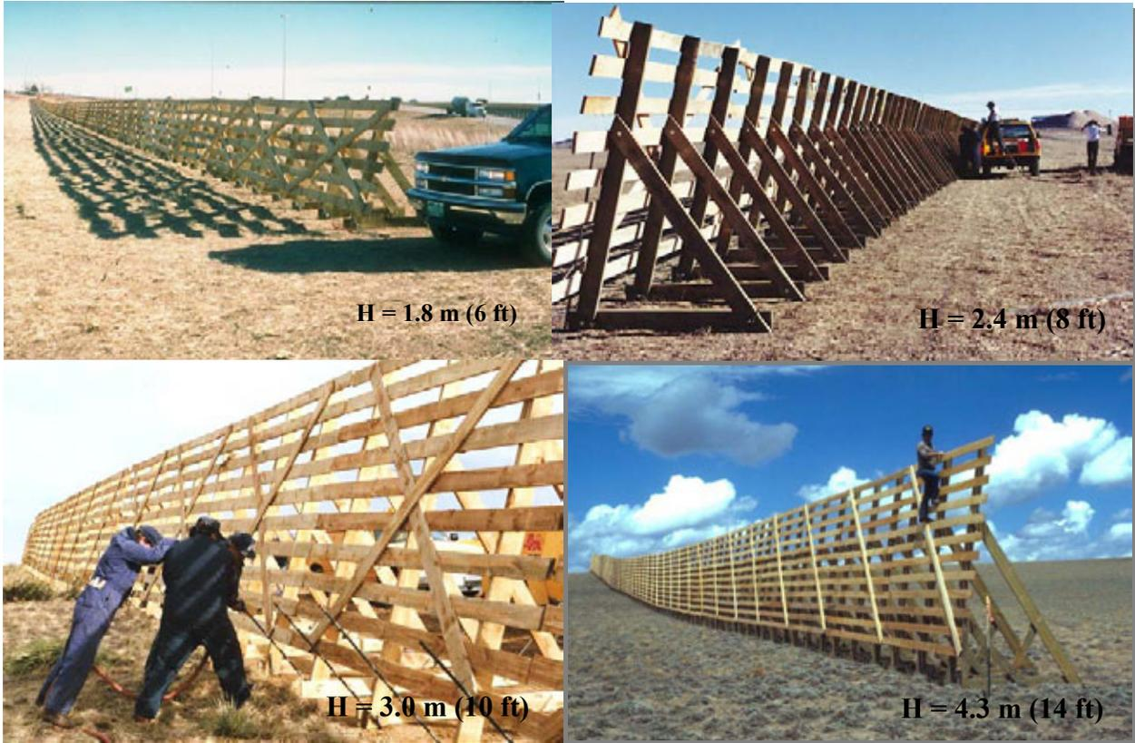
**Figure 6.6. Wyoming snow fence (lower right from Tabler, 1994).**
