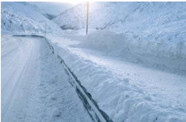
**Figure 5.15. Safety barrier prevents removal of roadside snowbanks.**
